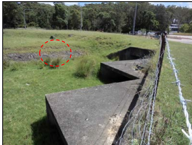
Figure 18: Photo showing both sets of culverts that discharge under Wyong Road/Tonkiss Street intersection. (Red circle identifies location of the northern culverts).
