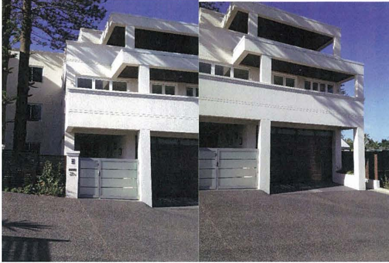
Photo 4 & 5 : 3-4 storey building behind No. 35 Hutton Rd
