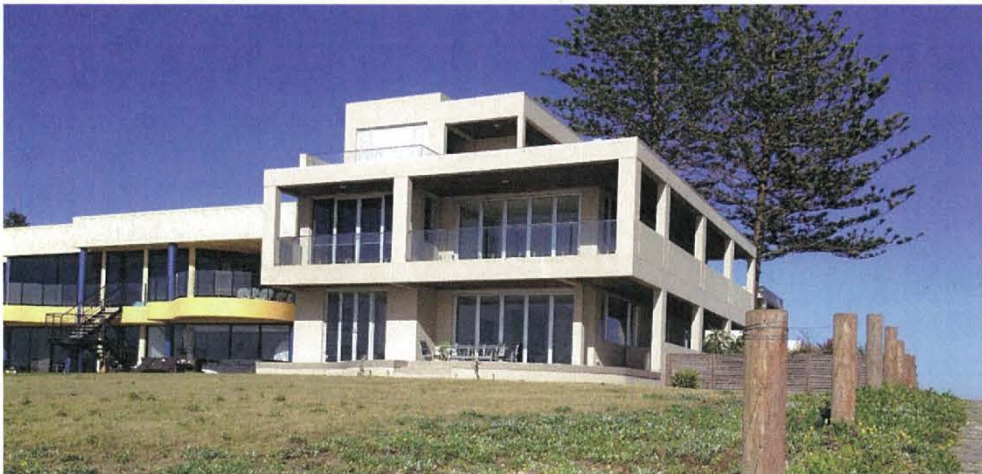
Photo 3: Dwelling at the rear of 35 Hutton Rd.
