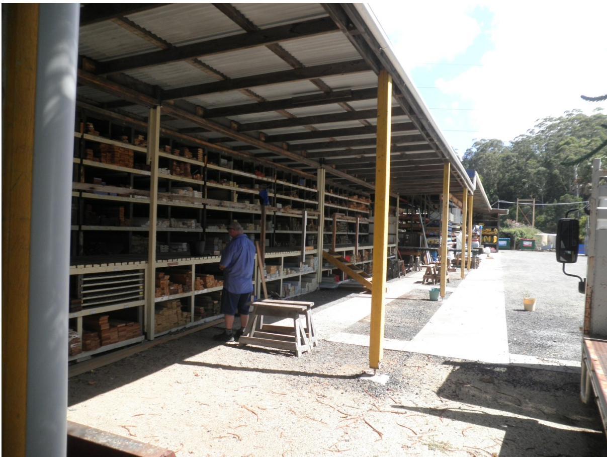
Figure 5: Awning structure and material storage on other side of Easement for Water Supply.
