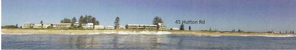
Photo 1: Looking North West. 2 & 3 storey buildings located south of Hargraves Street as they appear from the ocean.
