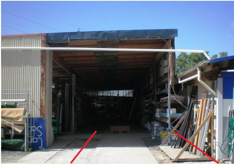
Figure 4: Recently constructed metal awning (easement for water superimposed in red)
