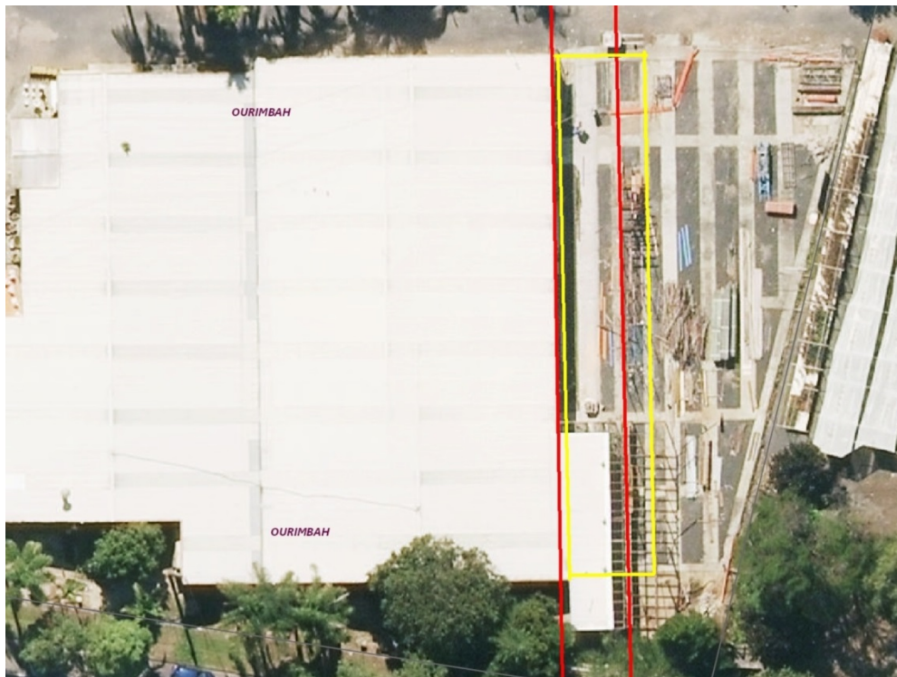
Figure 3: Early 2014 aerial view of site with water main easement (5.03 wide shown superimposed in red) minus approved shade structure and prior to unauthorized metal roof extensions (shown superimposed in yellow).
