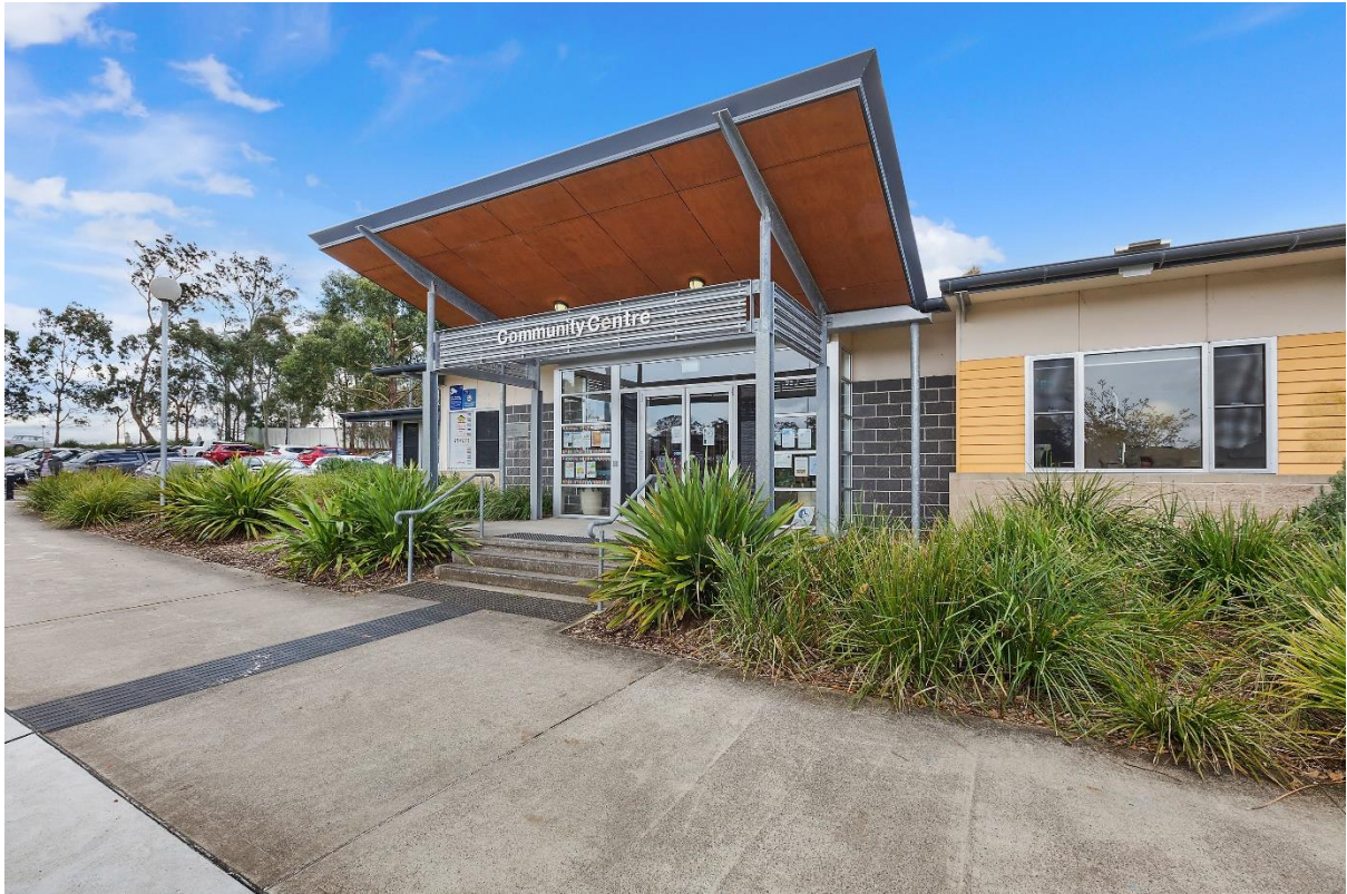
Front of the facility
