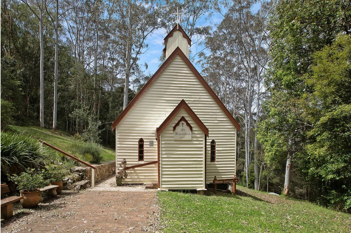
Front of the facility
