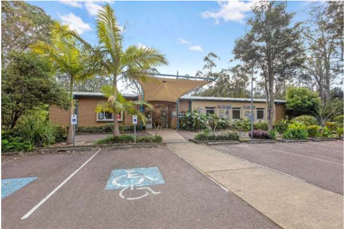
Front of the facility
