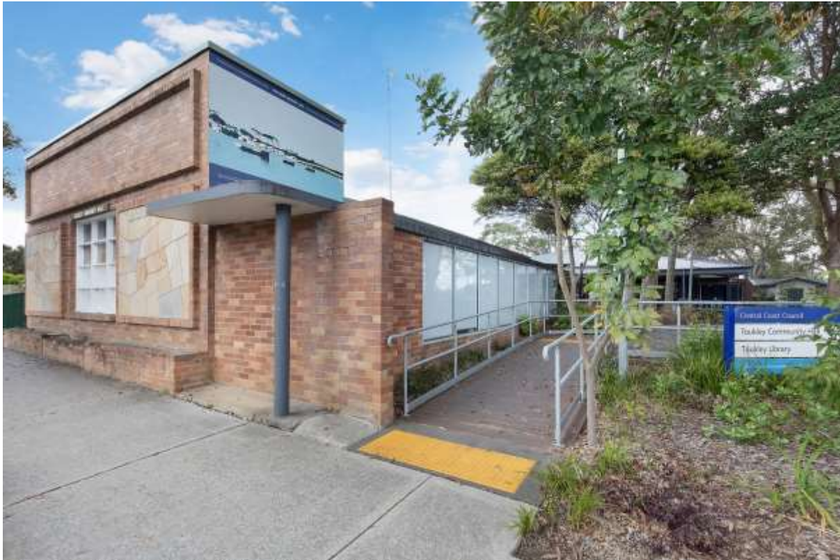
Front of the facility
