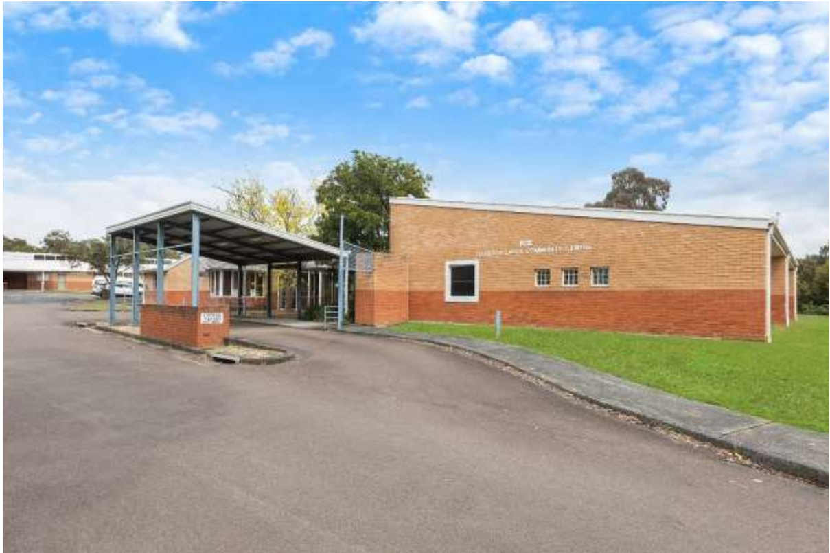
Front of the facility
