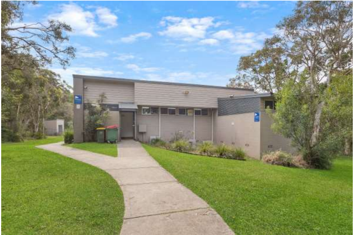
Front of the facility
