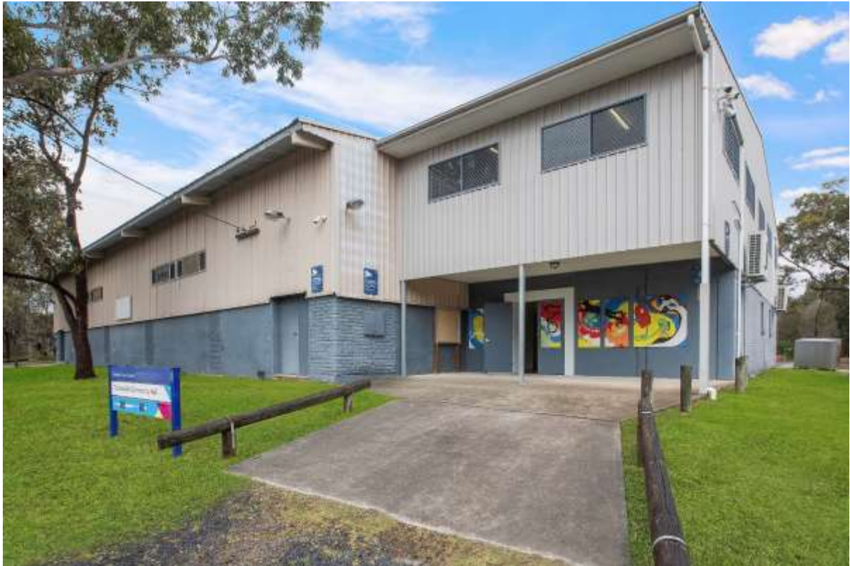
Front of the facility
