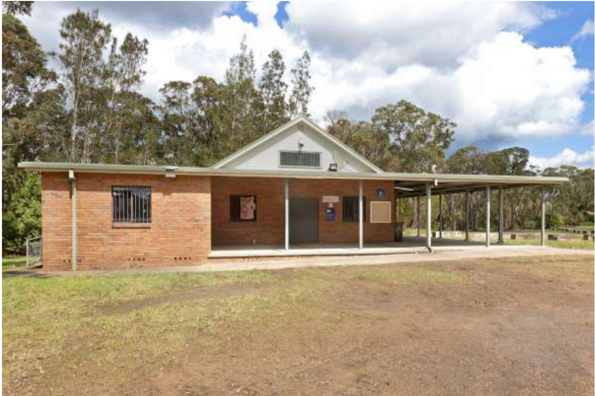
Front of the facility
