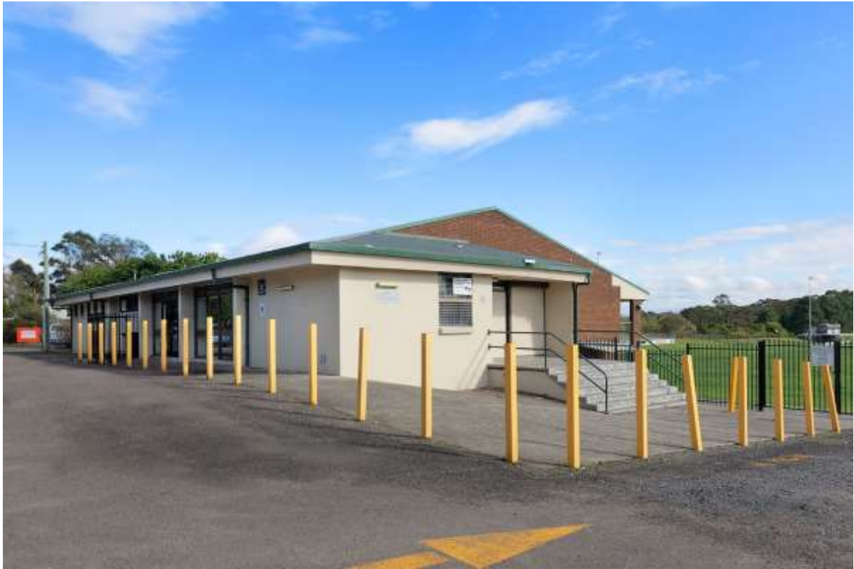
Front of the facility
