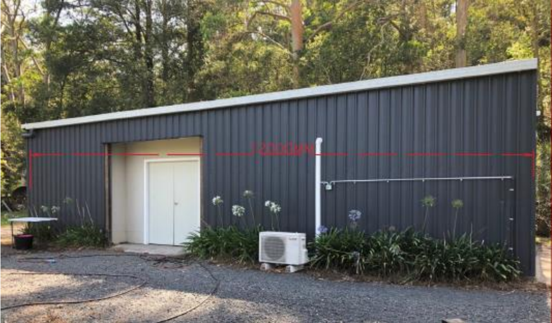
Figure 1 – Photo of existing shed currently being used to accommodate the dogs.
