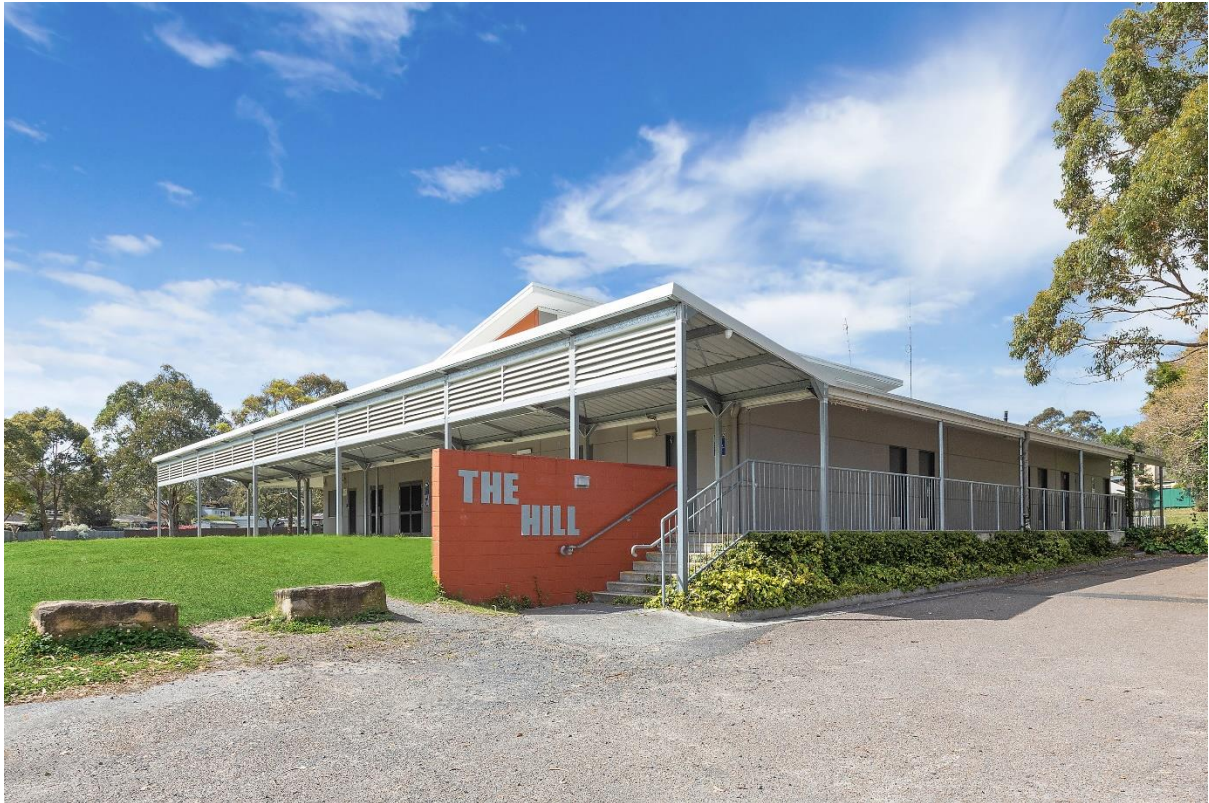
Front of the facility
