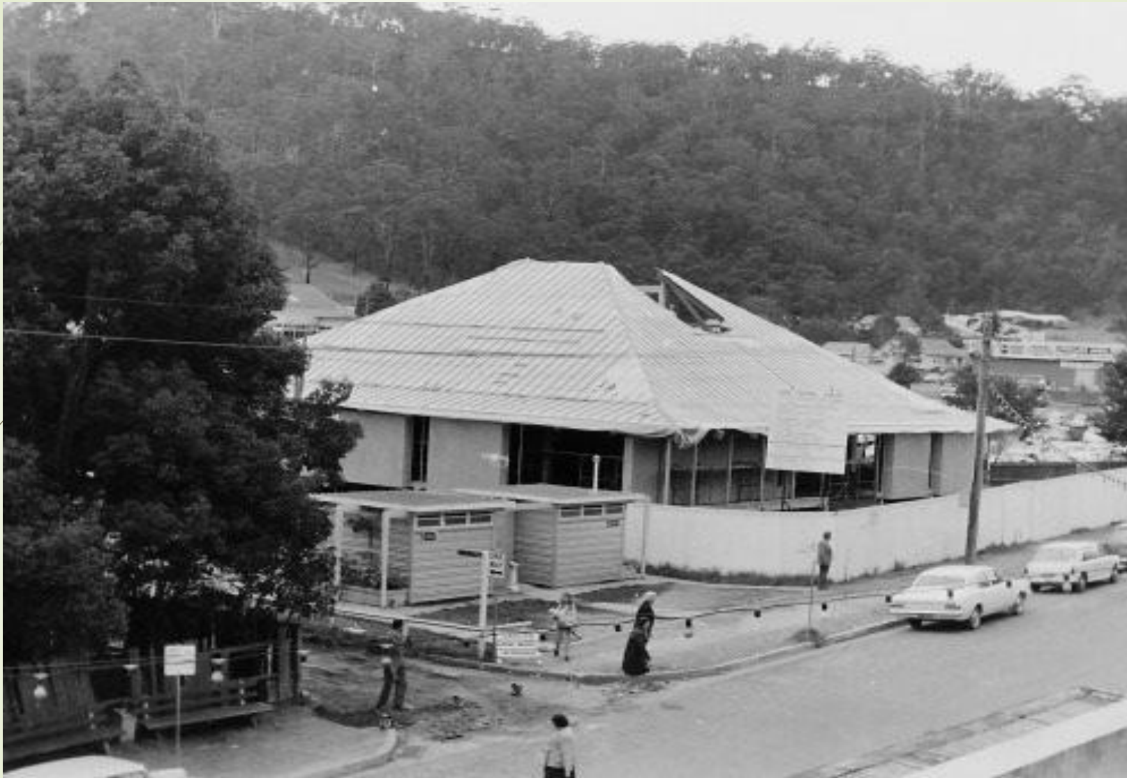
Gosford Library under construction in 1969.
