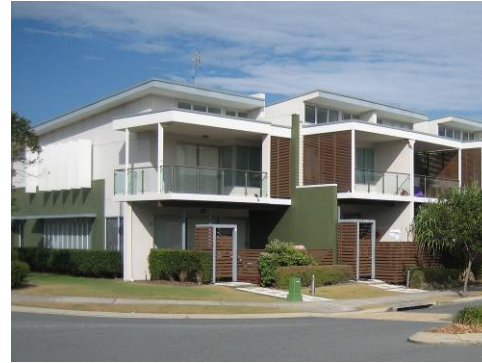
Photo 7: Town house, coastal example, NSW Coast
