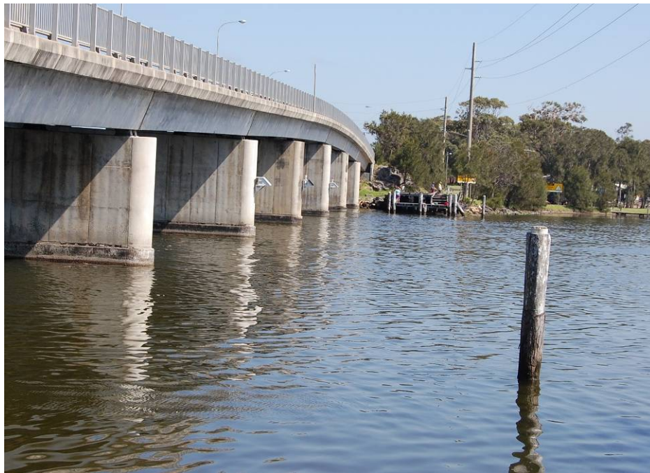
Photo 12: Toukley Bridge looking west
