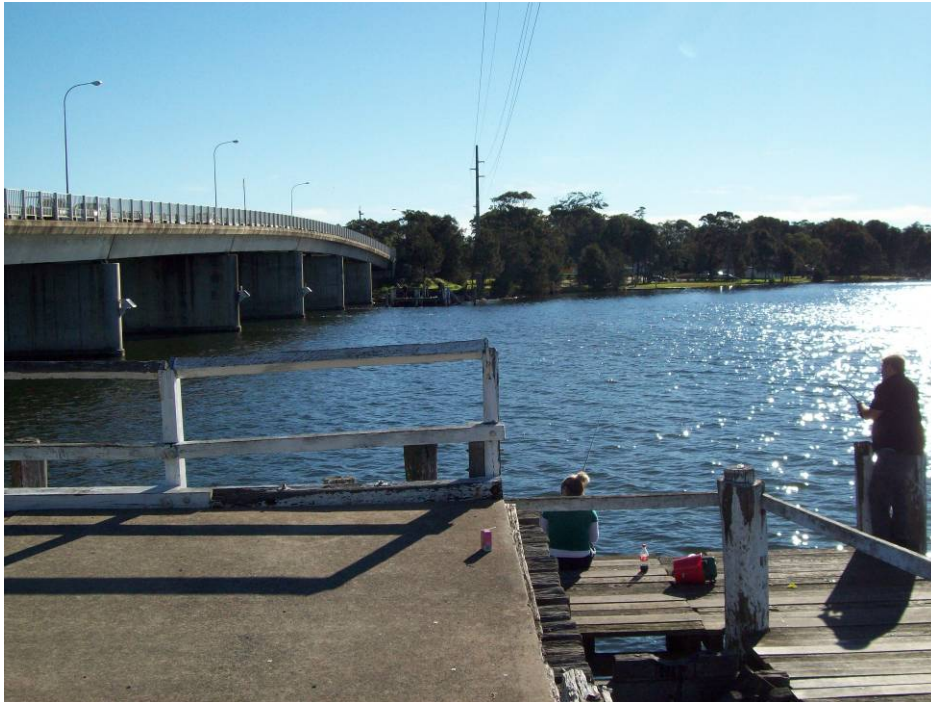
Photo 48: Wharf and old bridge remains, adjacent to Toukley Bridge
