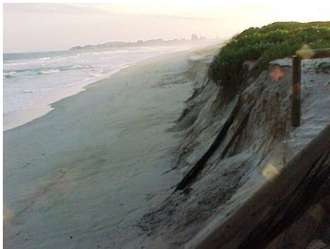
Photo 18: Coastal storm damage
