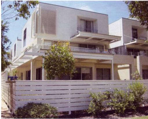
Photo 62: Example of three storey housing, Port Stephens
