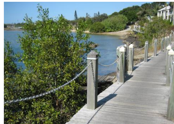
Photo 43: Coastal boardwalk, NSW Coast
