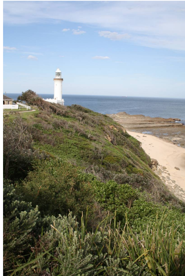
Photo 6: View of Norah Head Lighthouse and surrounds
