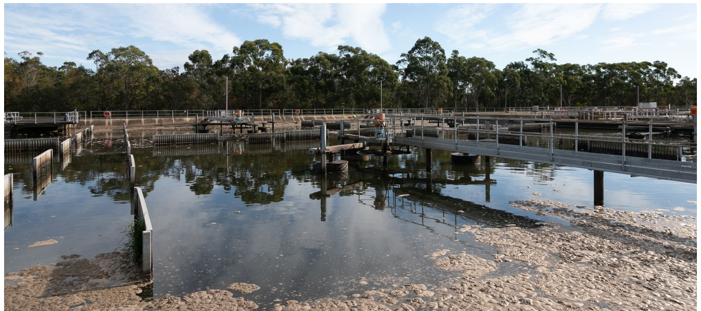
Figure 28 - Charmhaven Treatment Plant
