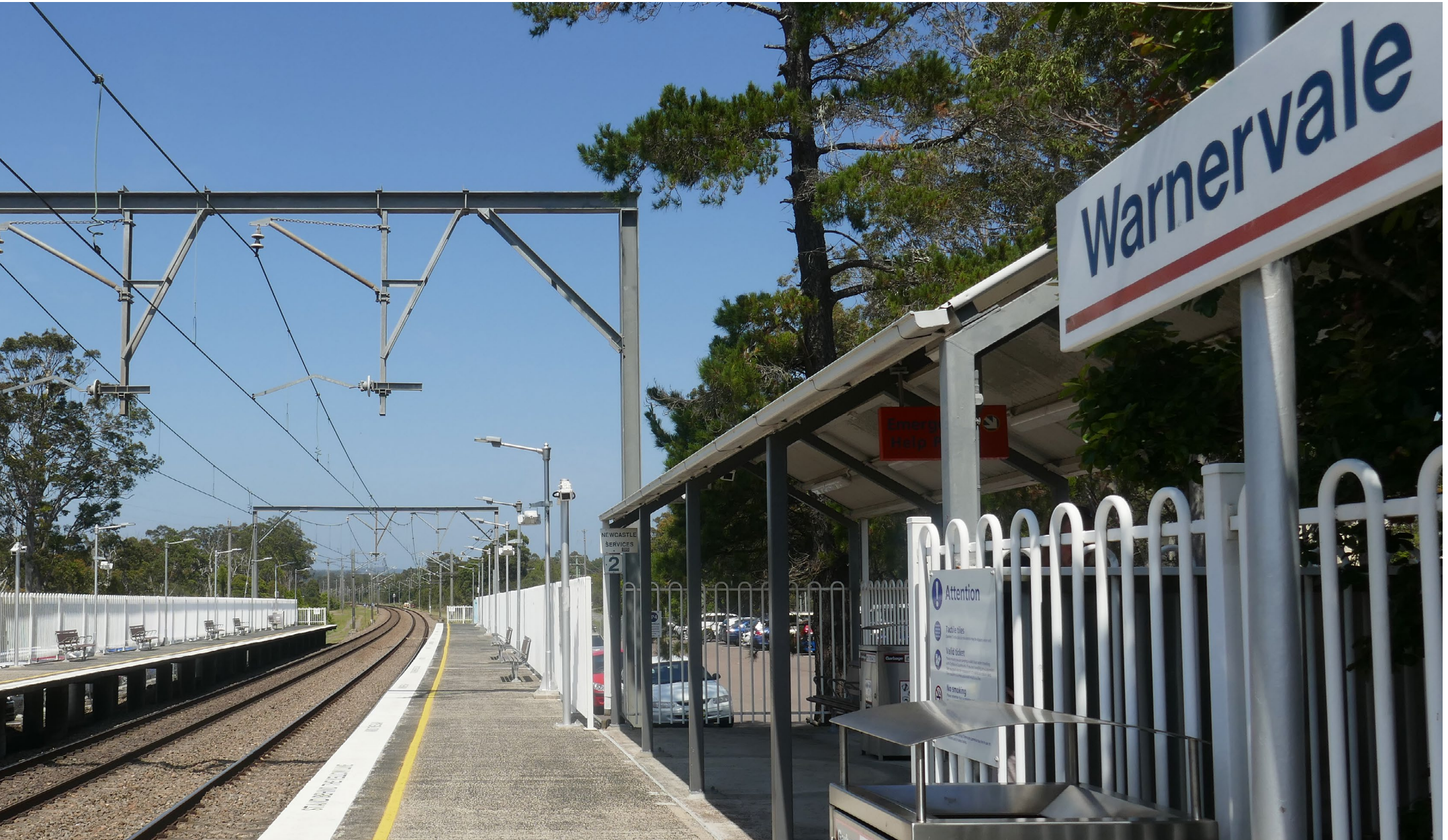
Figure 36 – Warnervale Railway Station
