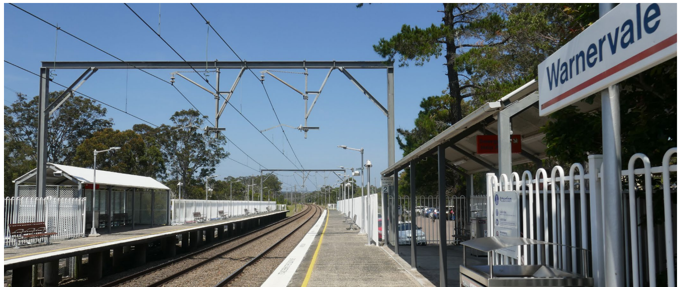
Figure 52 - Warnervale Railway Station
