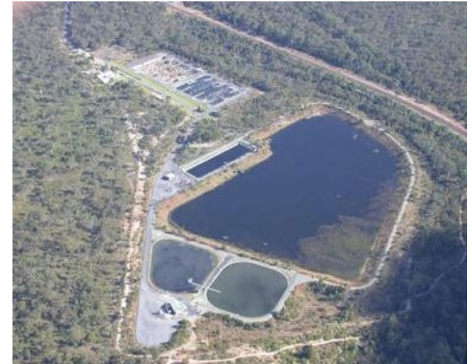
Figure 48 - Charmhaven Sewage Treatment Plant
