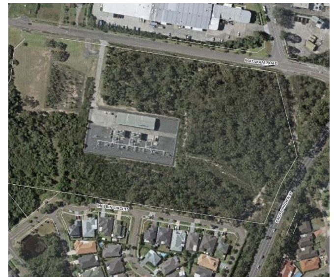
Figure 49 - Woongarra electricity substation
