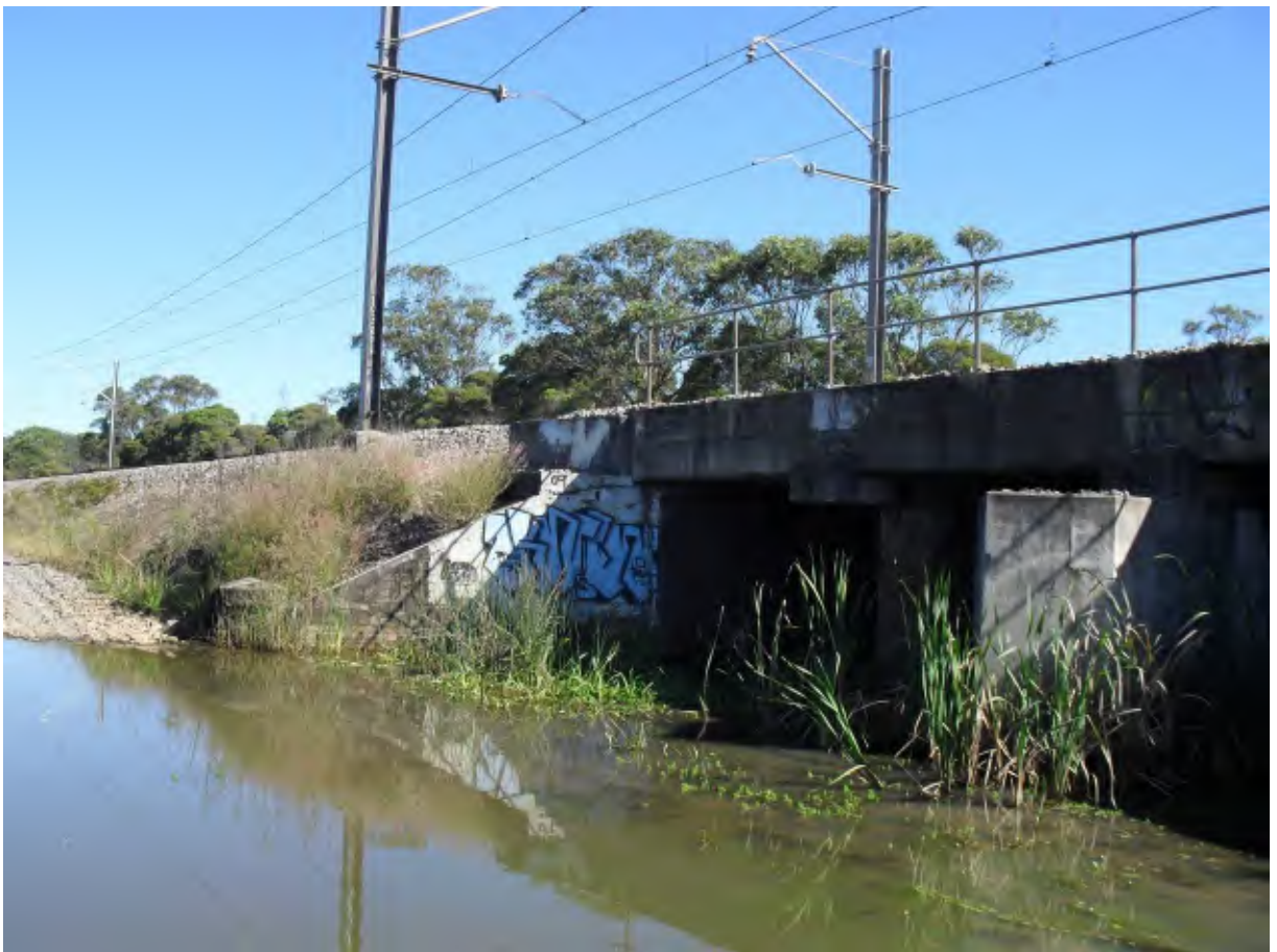
Central culvert inlet side, note brick central walls with triangular front edge
