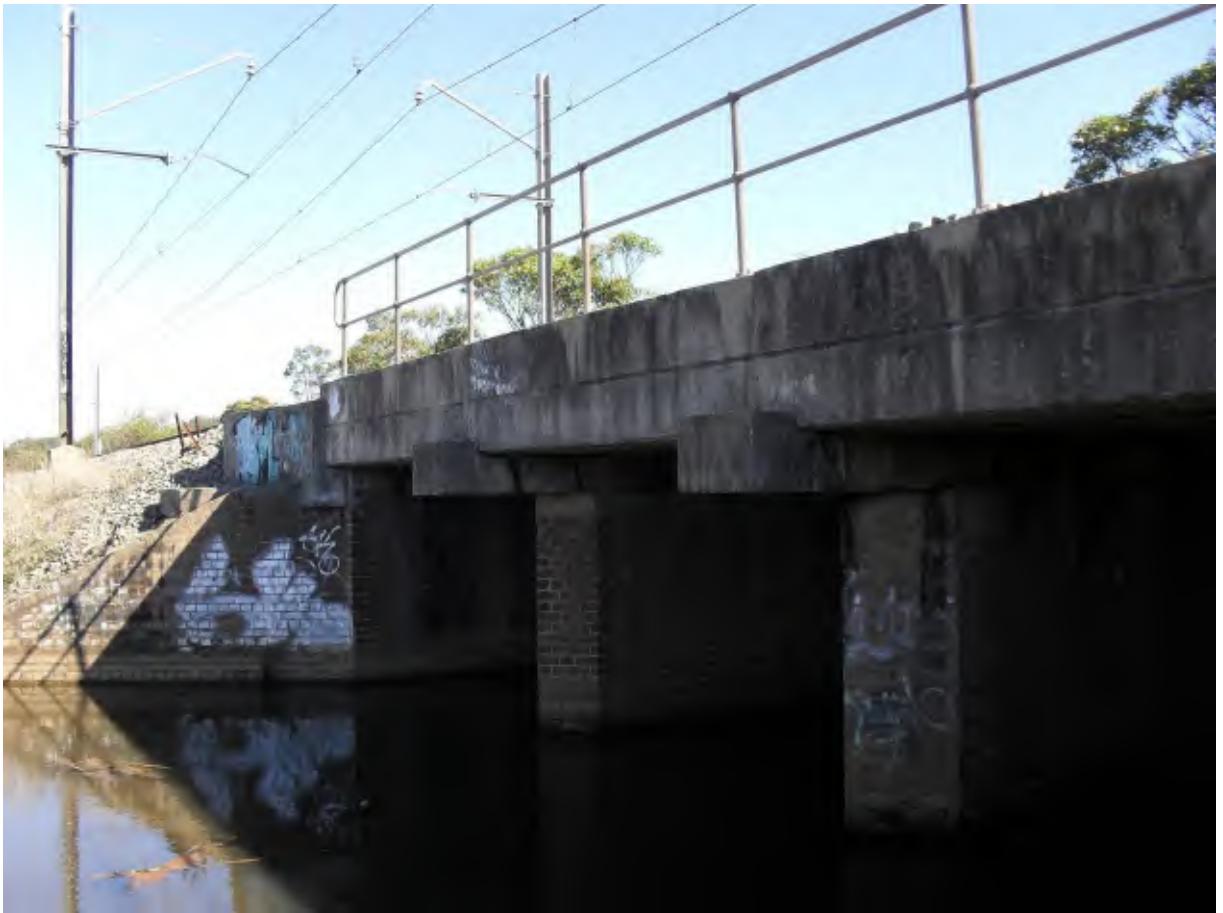
Central culvert inlet side, note brick central walls with triangular front edge
