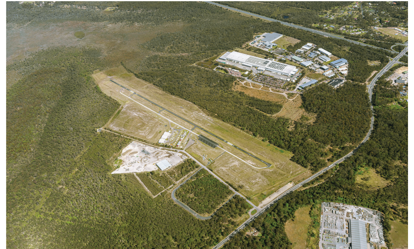
Aerial Photograph of the Central Coast Airport - 2024
