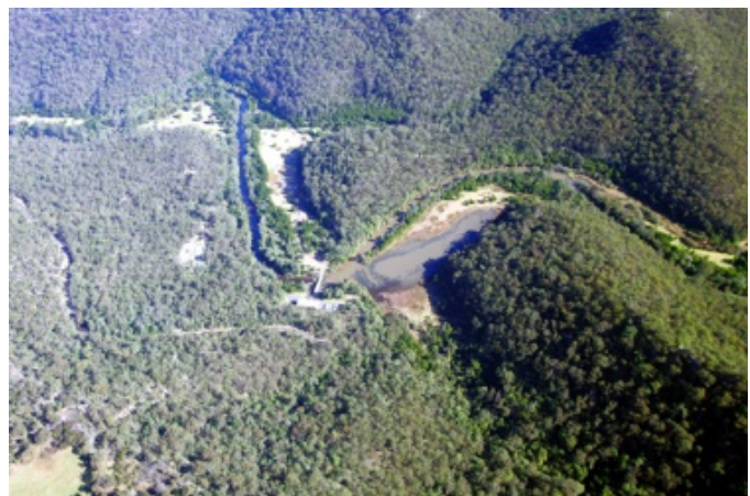
Mangrove Creek weir (Source: Central Coast Council)
