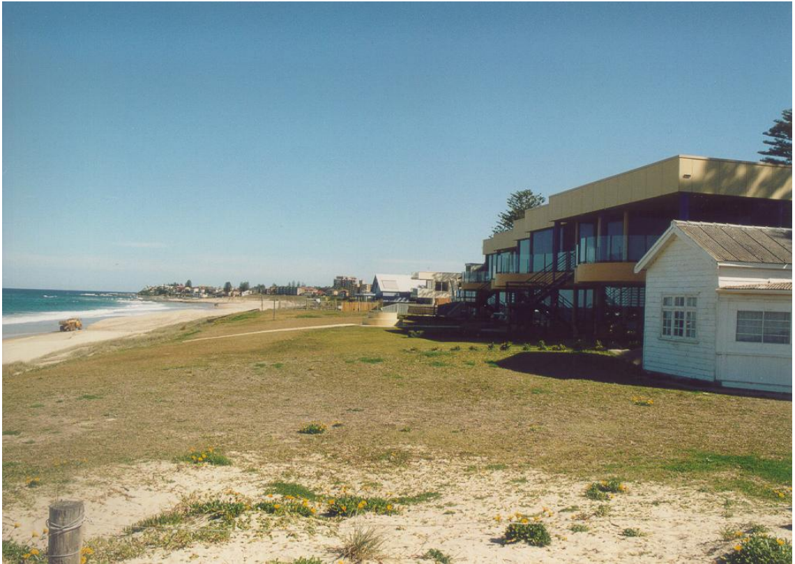
Figure B.13 – Typical view of North Entrance Beach, at Photogrammetry Block B
