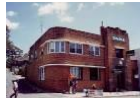
Former Rural Bank Pacific Highway
