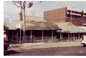
Police Station and Quarters Alison Road
