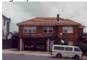
Brisbane Water Ambulance Station, Pacific Highway
