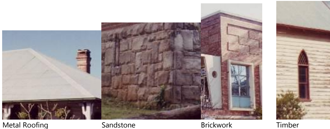
Figure 13 Examples of traditional materials found in the Wyong Town Centre heritage buildings
