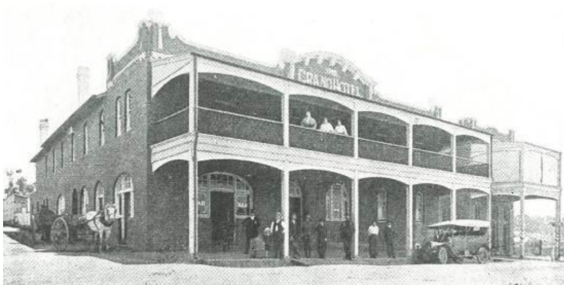
Figure 8 Historic photo of the Grand Hotel on the Pacific Highway (Source: Stinson)
