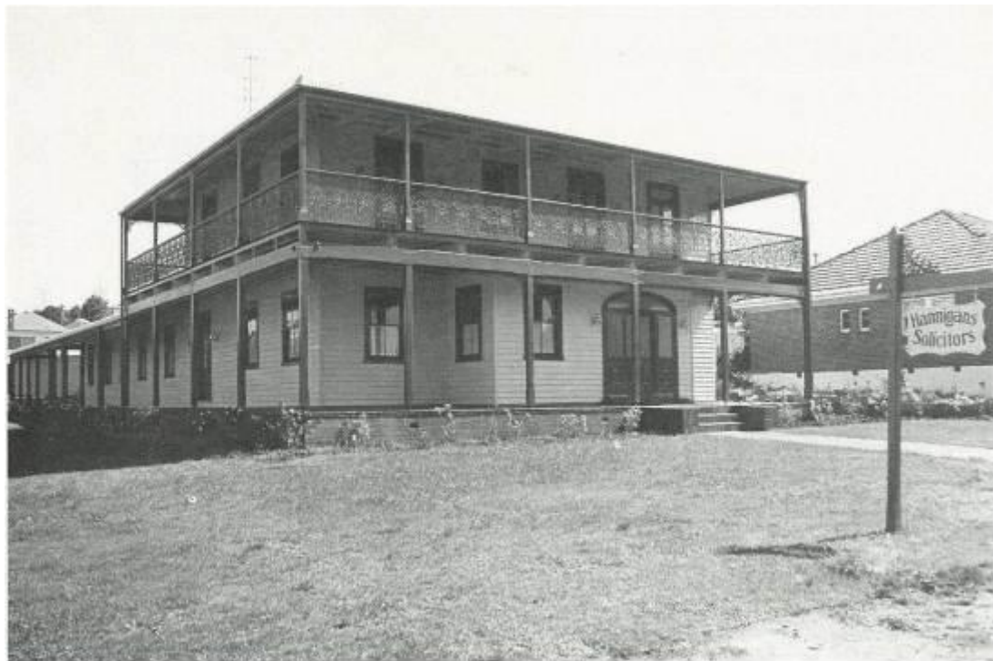
Figure 10 Solicitors' offices in an historic building on Margaret Street (Source: Stinson)
