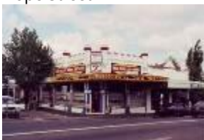
Shopping Complex Pacific Highway
