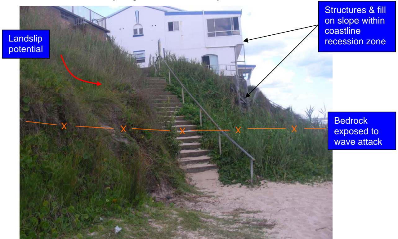
P3: Mechanism B – Soil & Fill Creep on Slopes. Map Area G6: Land instability occurring in fill & soil slope above Patonga Claystone bedrock in coastline recession zone.
