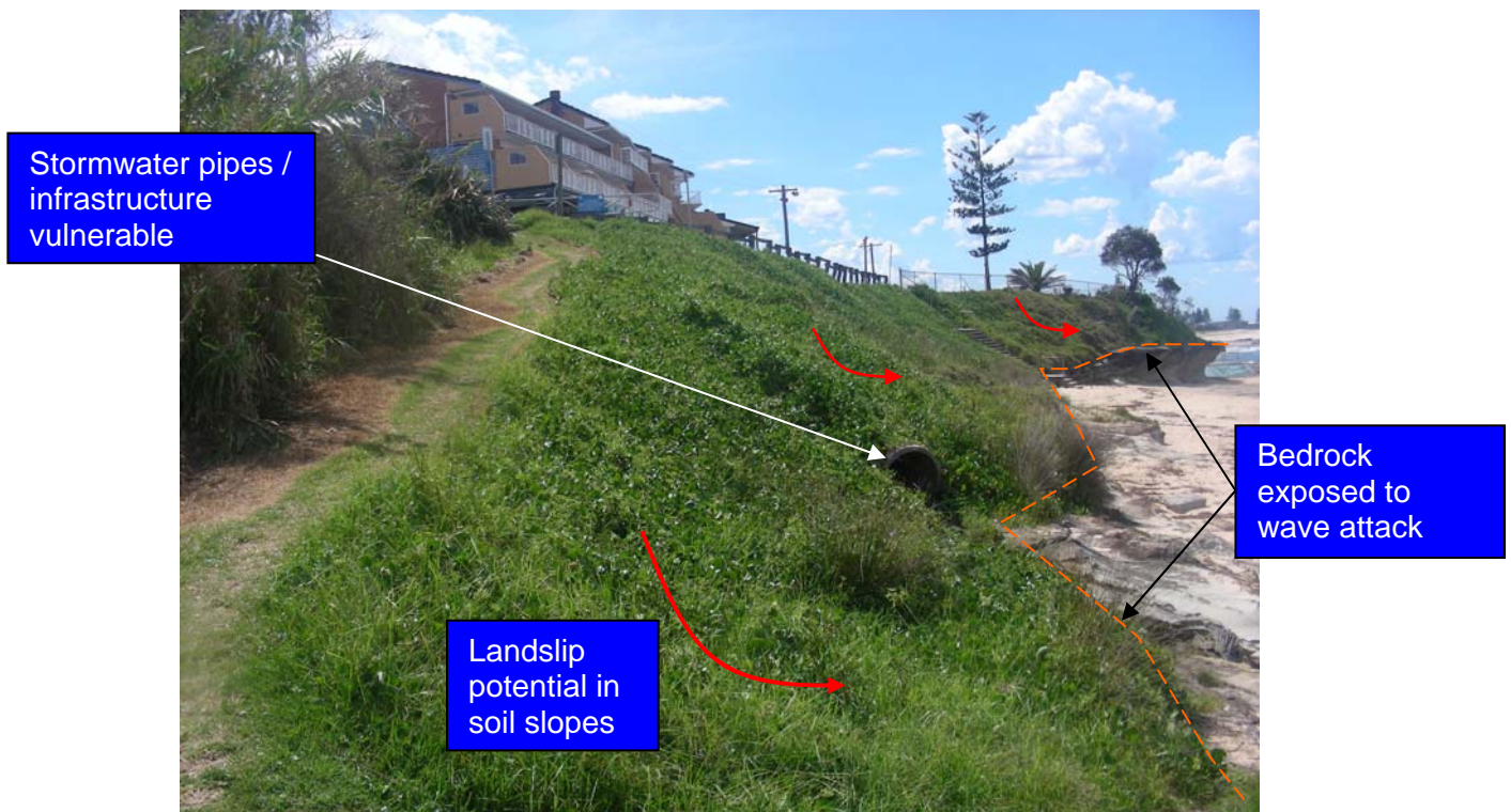
P4: Mechanism B – Soil & Fill Creep on Slopes. Map Area G6: Land instability occurring in fill & soil slope above Patonga Claystone bedrock in coastline recession zone.
