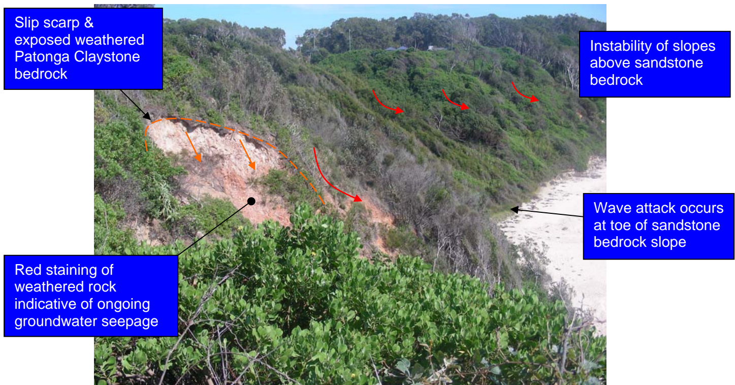
P14: Mechanism E – Instability of Weathered Rock / Soil Slope. Map Area G12: Patonga Claystone weathered rock / residual soil slope instability, over Tuggerah Formation in coastline recession zone.
