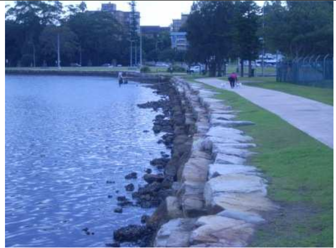
Photo 26: Point Frederick seawall looking north. (W69)
