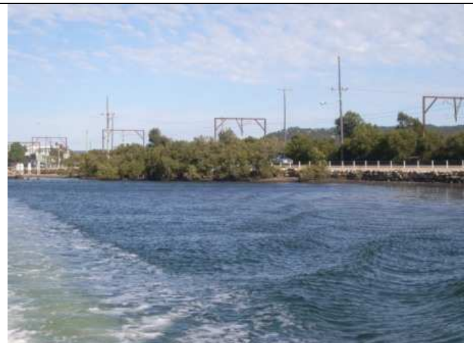
Photo 42: Brisbane Water Drive causeway adjacent to railway line (looking west). (W11, W12, R35)
