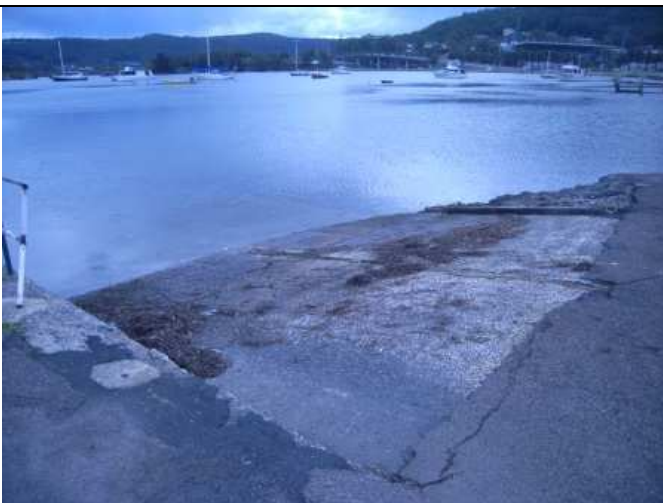
Photo 5: Boat ramp next to Iguana Joe's, Gosford. (P48, R31)
