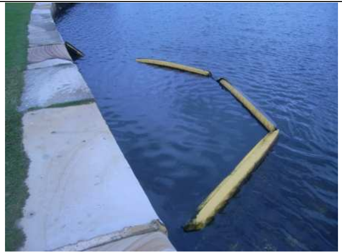
Photo 4: Stormwater traps along Gosford foreshore. (W27)
