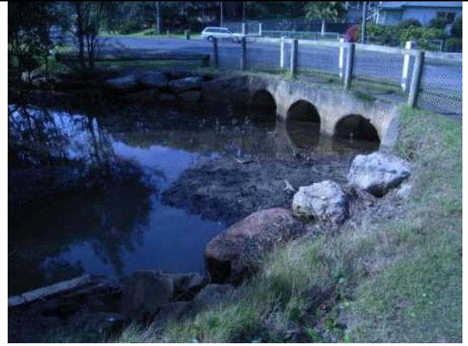
Photo 34: RSL Creek culvert into Hardys Bay. (W23)
