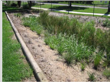
Example: Sediment trap as part of a stormwater treatment train
