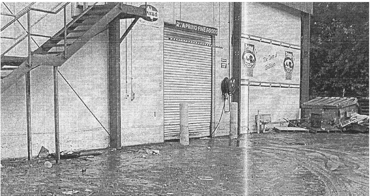
Figure 6-4 March 2002.B – Photograph Looking at Coorumbine Creek near Primo Fine Foods
