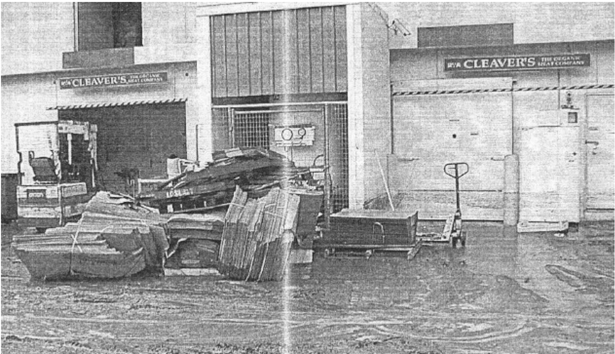
Figure 6-3 March 2002.A – Photograph Looking at Jusfrute Dr from Coorumbine Creek
