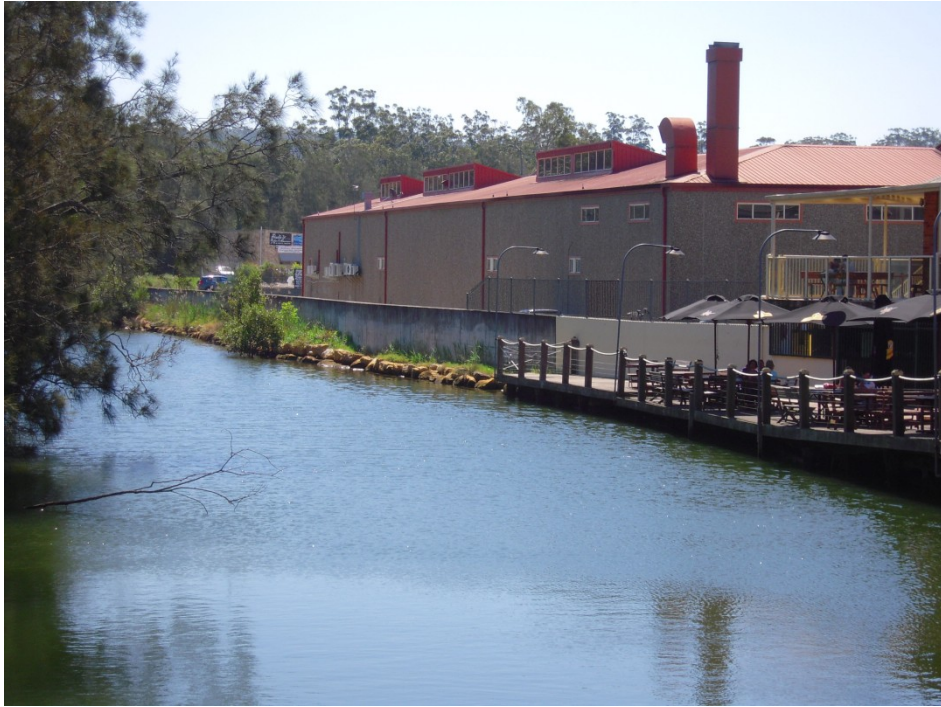
Photograph 7: Concrete levee, Erina Creek.
