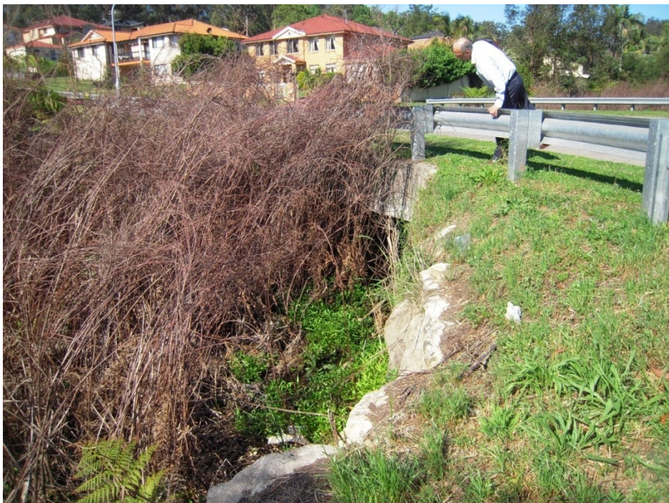
Photograph 10: Worthing Road Creek - obstructed culvert at Jessie Hurley Drive near Stringybark Close
