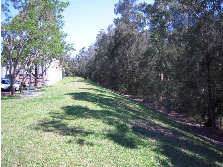
Photograph 5: Earthen levee, west of Bonnal Road, looking downstream
