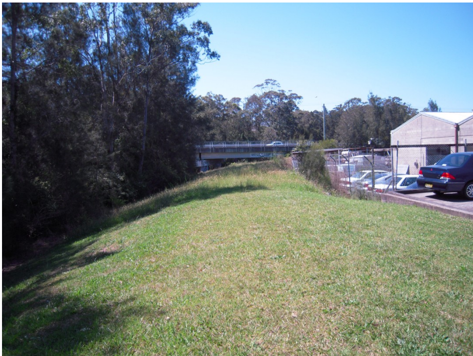
Photograph 6: Earthen levee, west of Bonnal Road, looking upstream
