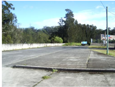
PHOTOGRAPH 3: Concrete levee preventing inflow at Bonnal Road
