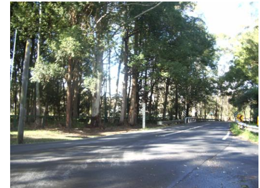
PHOTOGRAPH 8: Carlton Road bridge over Erina Creek showing flood depth indicator on left.
