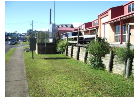
PHOTOGRAPH 7: Buildings and services built on elevated pads above the level of flood waters.
