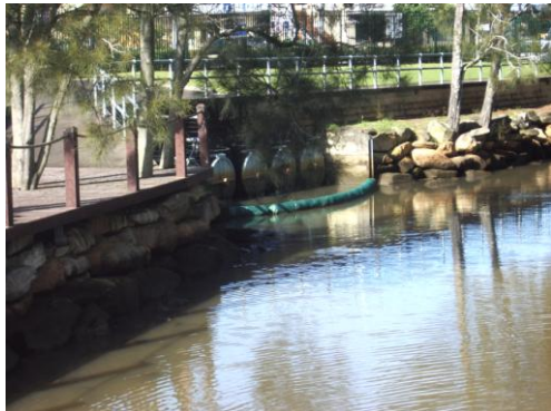
PHOTOGRAPH 2: Flap gated culverts preventing high water levels in Erina Creek from affecting upstream properties near Karalta Rd.
