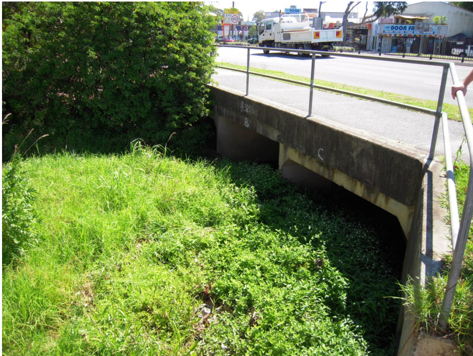
Photograph 9: Nunns Creek – triple box culvert at the Central Coast Highway
