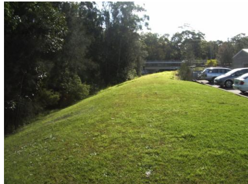
PHOTOGRAPH 4: View to Barralong Road bridge along earthen levee protecting industrial properties on the right of the photo.
