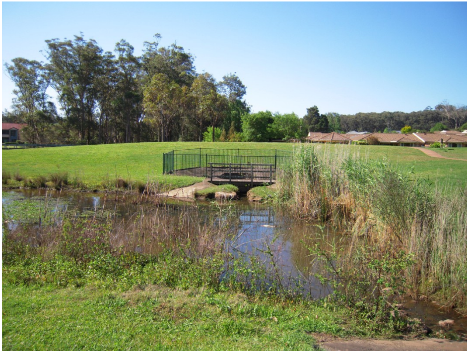
Photograph 8: Retarding basin at Worthing Road Creek
