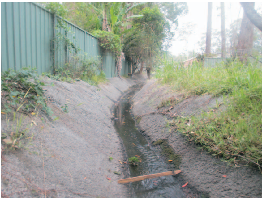
Concrete-lined open channel near Water Street, Kincumber
