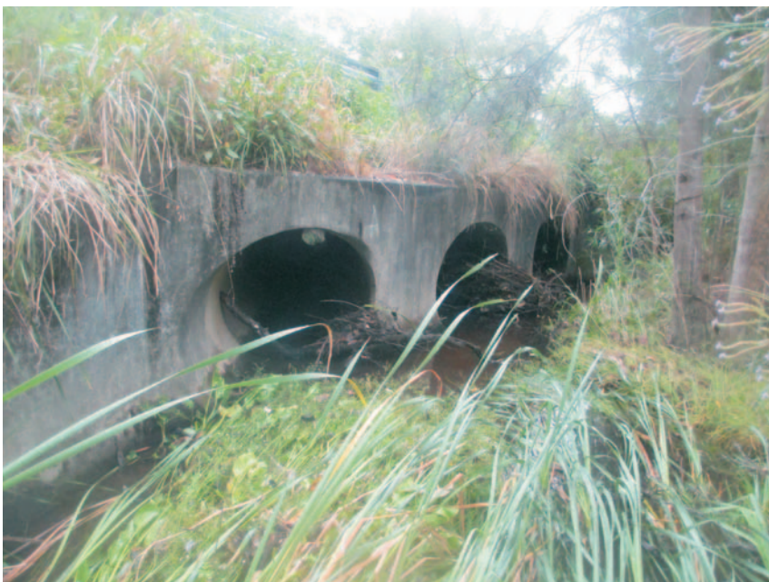
Large culverts crossing Empire Bay Drive near Bundaleer Crescent, Bensville
