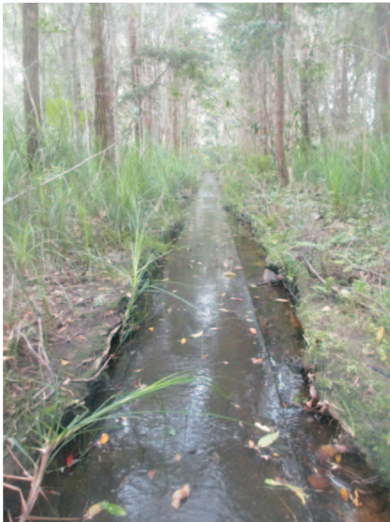
Concrete-lined flow path between Cullens Road and Water Street, Kincumber
