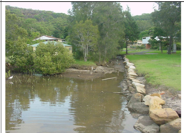
Stormwater drainage channel
