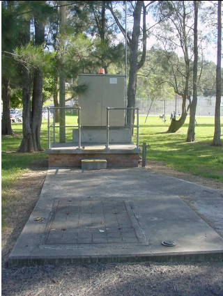
Waste water pumping station
