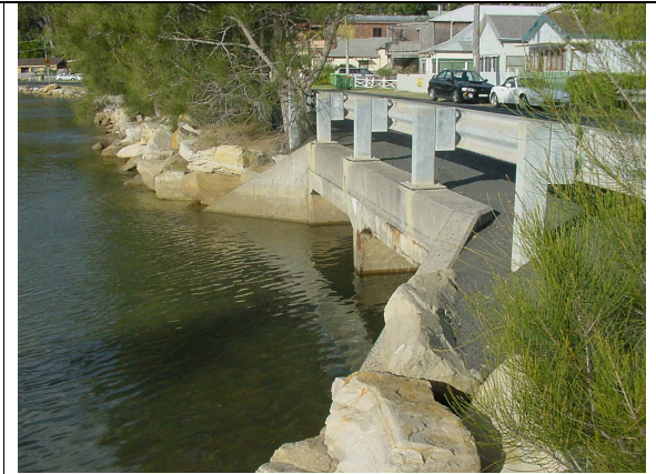
Pretty Beach Road culverts
