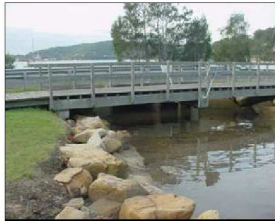
Pretty Beach Road Culverts
