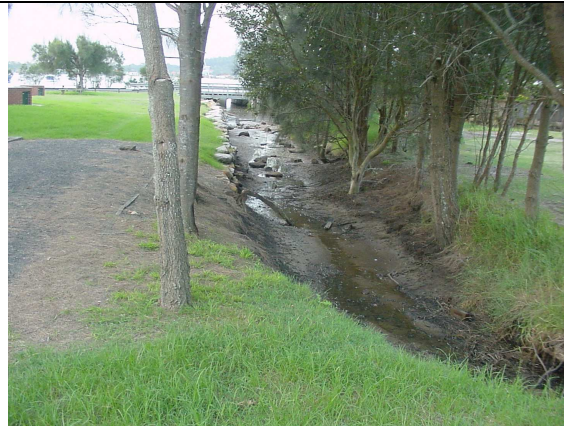
Channel carrying stormwater pipe flow from Turo Creek Catchment
