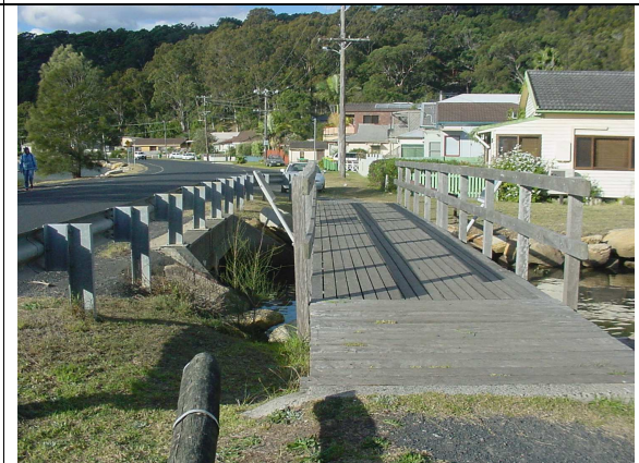
Pedestrian Bridge, Pretty Beach Road
