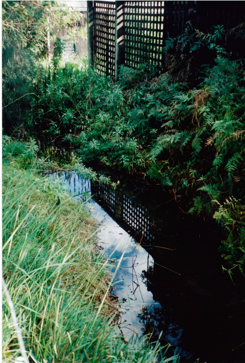
Open Drain behind houses on Rickard Rd
