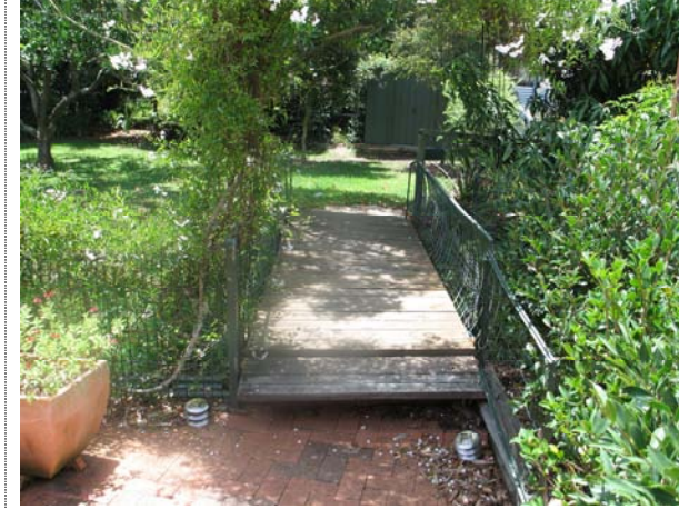
Photo 27: Bridge in 48 Venice Rd. Looking east
