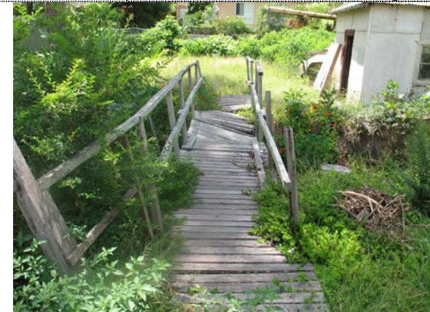
Photo 18: Bridge in 44 Venice Rd, looking East
