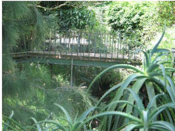
Photo 25: Bridge in 48 Venice Rd - Photo taken from 46 Venice Rd from the left bank of the creek, looking upstream
