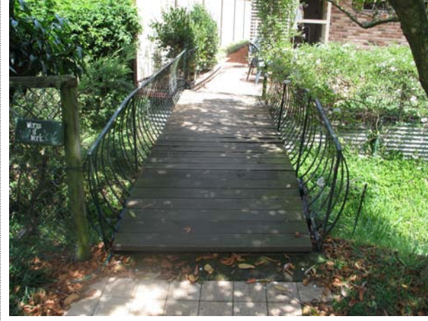
Photo 26: Bridge in 48 Venice Rd. Looking west
