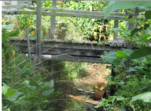
Photo 17: Bridge in 44 Venice Rd, looking from downstream
