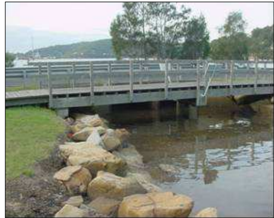
Pretty Beach Road Culverts
