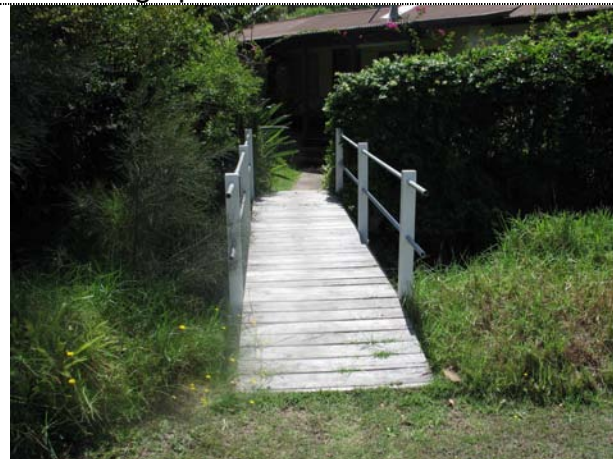
Photo 6: Bridge in 38 Venice Rd - Looking east, showing the bridge deck and railing
