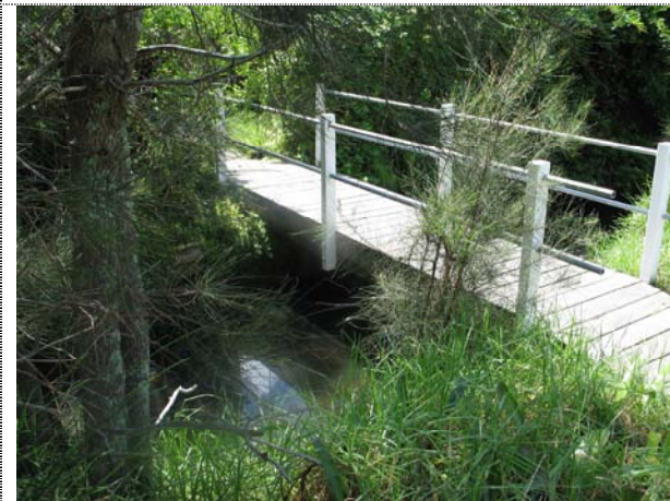
Photo 7: Bridge in 38 Venice Rd - Taken from downstream, left bank
