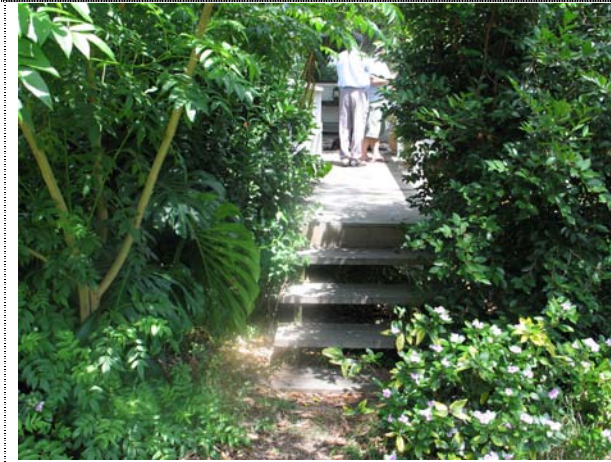
Photo 21: Deck-Bridge in 46 Venice Rd. Seen from the eastern side of Turo Creek, looking west.
