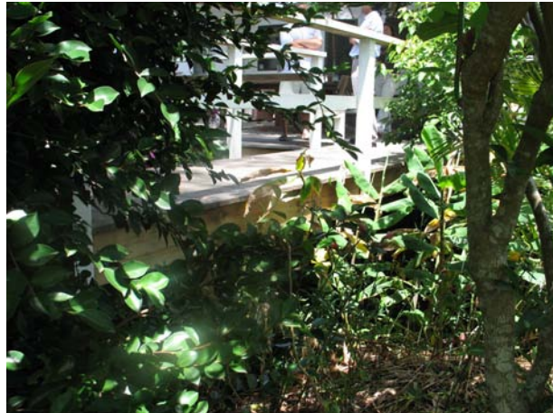
Photo 22: Deck-Bridge in 46 Venice Rd. Seen from the eastern side of Turo Creek, looking west showing downstream side of the bridge. 46 Venice Rd is the most heavily vegetated property with a large gum tree in the left bank of Turo Creek.
