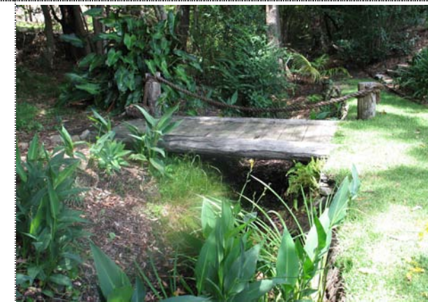
Photo 31: Downstream edge of the creek confinement in 50 Venice Rd.
