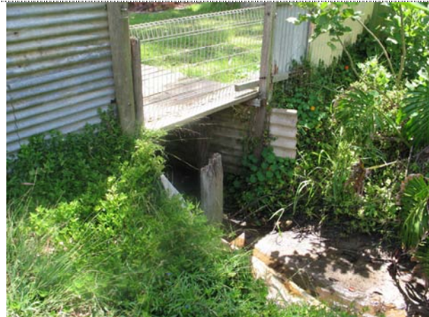
Photo 16: Creek Confinement in 42 Venice Rd, looking from upstream left bank.
