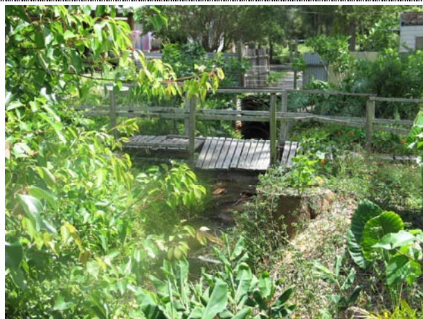
Photo 19: Bridge in 44 Venice Rd, View from deck-bridge of 46 Venice Rd (looking down-stream))
