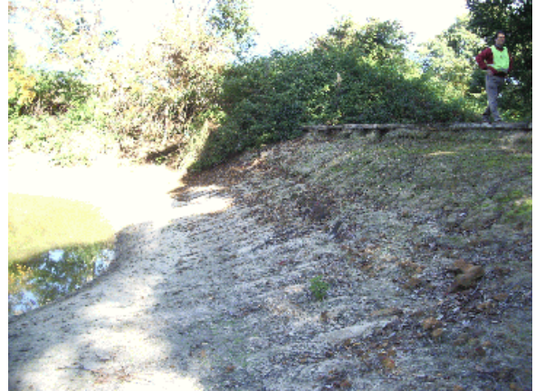
Photo 27: Dam Wall of Basin No. 3
