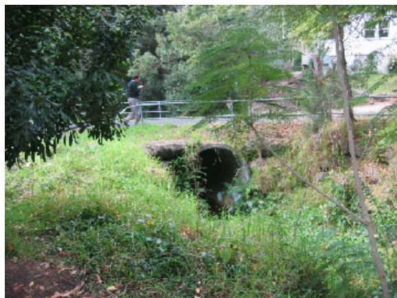
Photo 4: Fraser Road culvert looking upstream.
