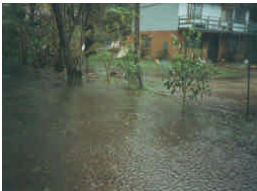
Photo 9: Upstream of Noble Road bridge - July 1988.
