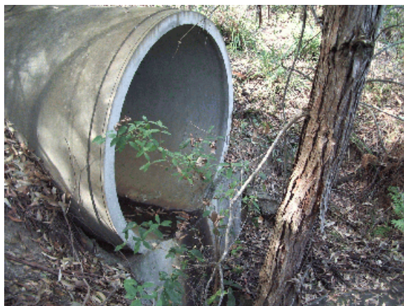
Photo 21: 1800 mm outlet pipe under Wards Hill Road
