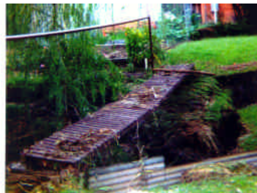
Photo 8: Rear of 45 Fraser Road - February 1990.
