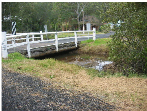
Photo 1: Noble Road Bridge looking upstream.
