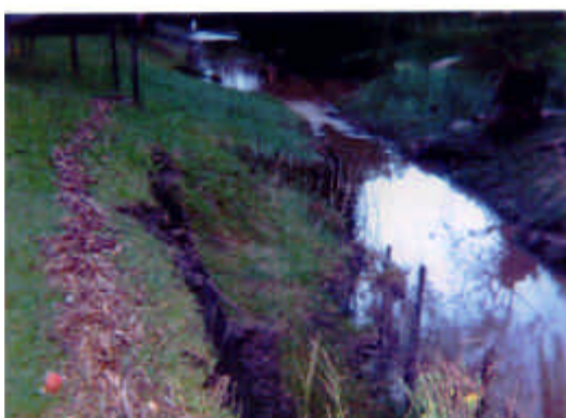
Photo 7: Rear of 45 Fraser Road - February 1990.
