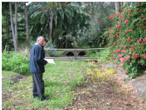
Photo 2: Twin 900 mm diameter pipe outlet into Mudflat Creek at rear of 57 Fraser Road. Note siltation covering half of pipes at the outlet.
