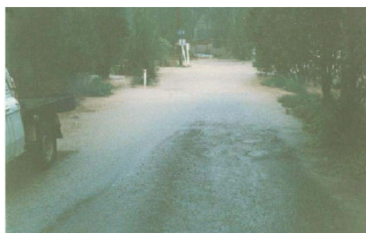
Photo 17: At Fraser Road culvert. View looking south.
