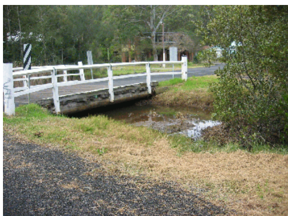
Photo 1: Noble Road Bridge looking upstream.
