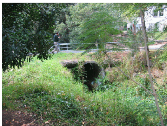
Photo 4: Fraser Road culvert looking upstream.
