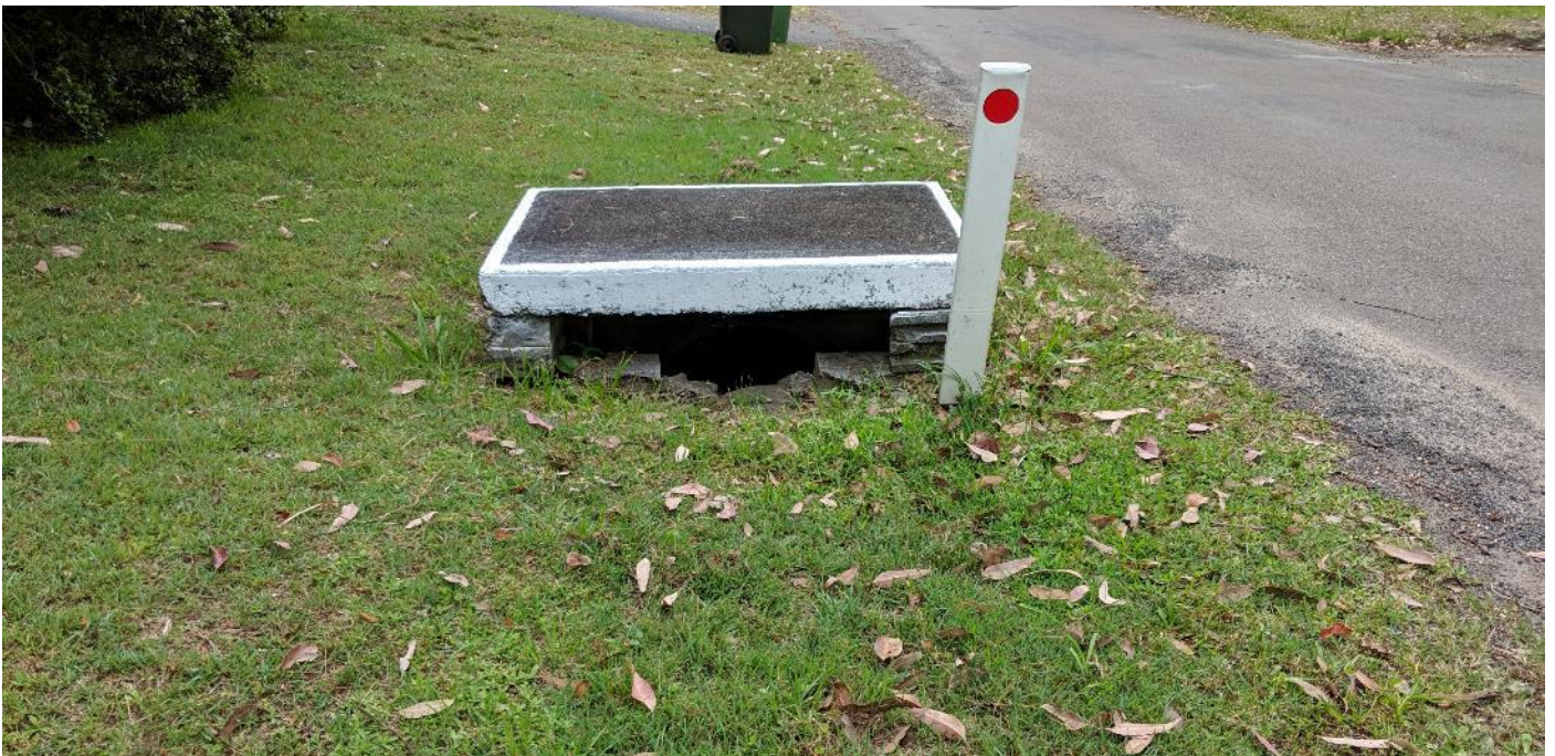
Empire Bay – typical letterbox style inlet pit
