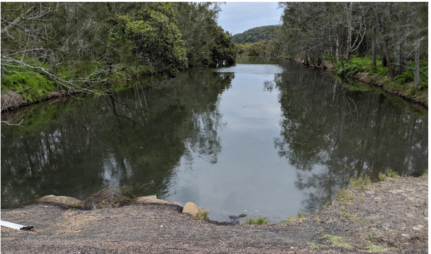
Davistown – channel at Malinya Road looking west
