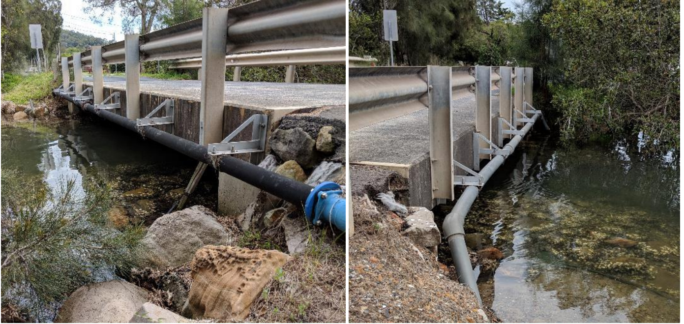
Davistown – Morton Crescent bridge downstream / upstream
