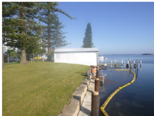
The Entrance foreshore improvement works
