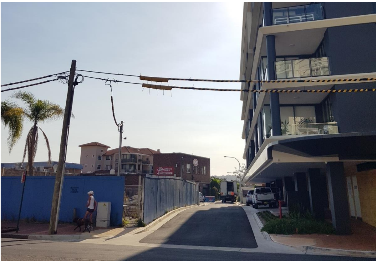
Figure 5 – Atlantis development interface across unnamed lane looking generally north east. The subject land is to the left of the unnamed laneway.
