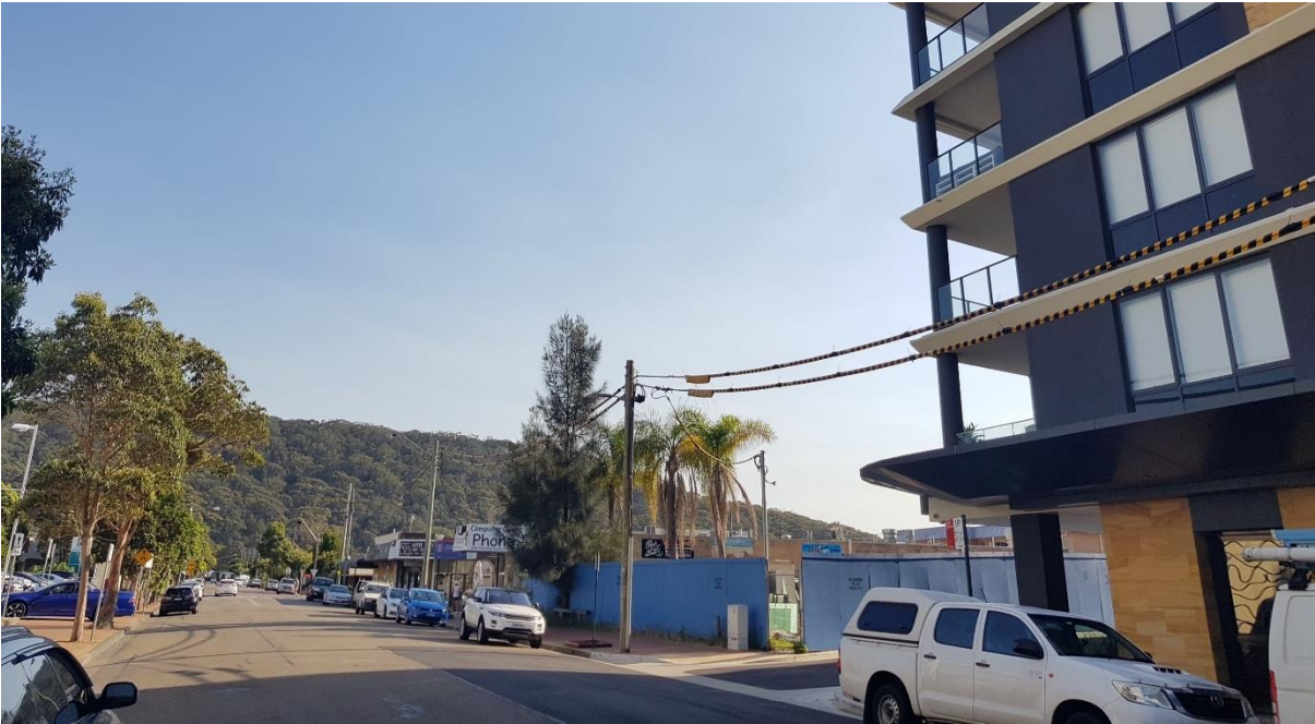
Figure 4 – Site from Memorial Avenue looking generally north
