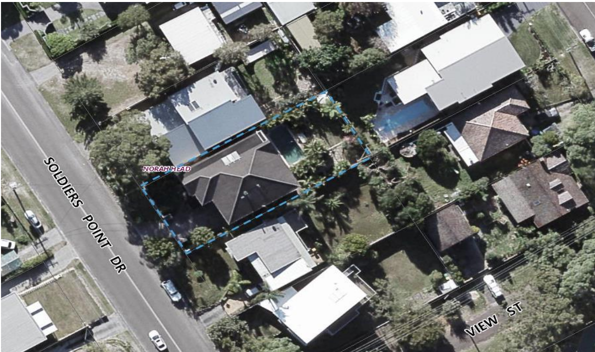
Figure 2: Closer aerial photo of the site and surrounds
