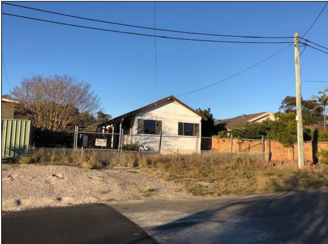
Figure 2 – View of the site from Clifford Street
