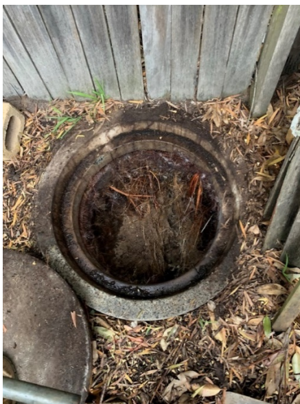
Figure 3: Tree roots in a sewer manhole in Council's sewer system
