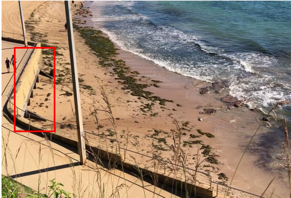
Figure 1 Seven drains outlet onto the southern end of Terrigal Beach on 24 April, location of the drainage outlets indicated by red rectangle.
