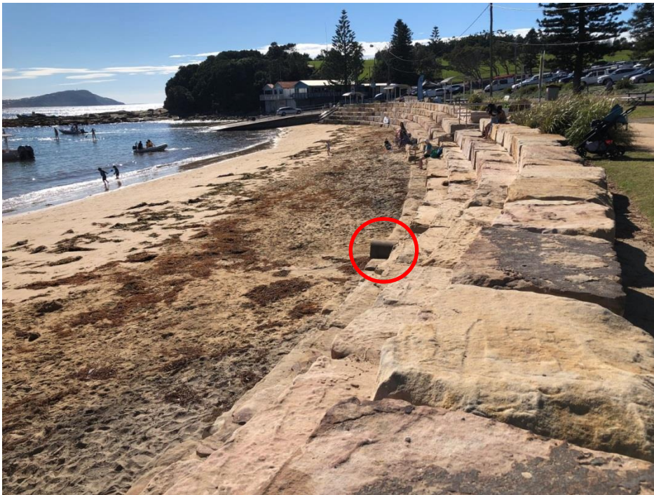
Figure 2 Stormwater outlet (indicated by a red circle) at The Haven on 26 April 2019
