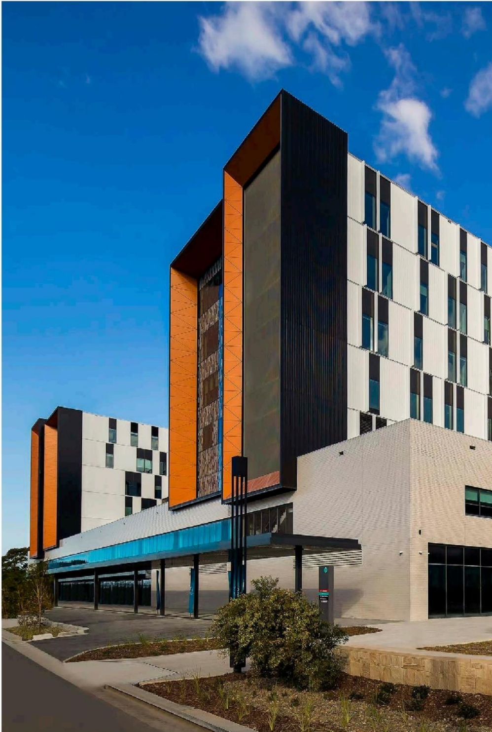
NORTHERN BEACHES HOSPITAL Photo credit: Ministry of Health
