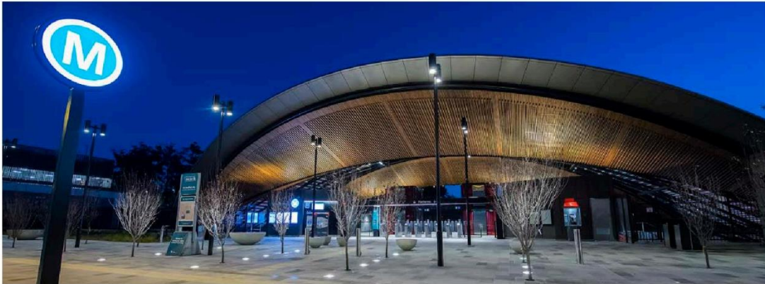
CHERRYBROOK METRO STATION Photo credit: Sydney Metro
