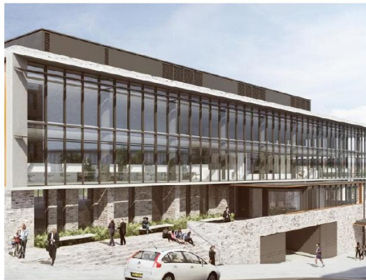
The new Gosford ATO office, corner of Mann Street and Georgiana Terrace, Gosford
