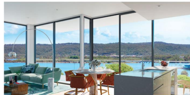
The Albany, Point Frederick (currently under construction) Source: http://richardrookes.com.au/project/the-albany-apartments/
