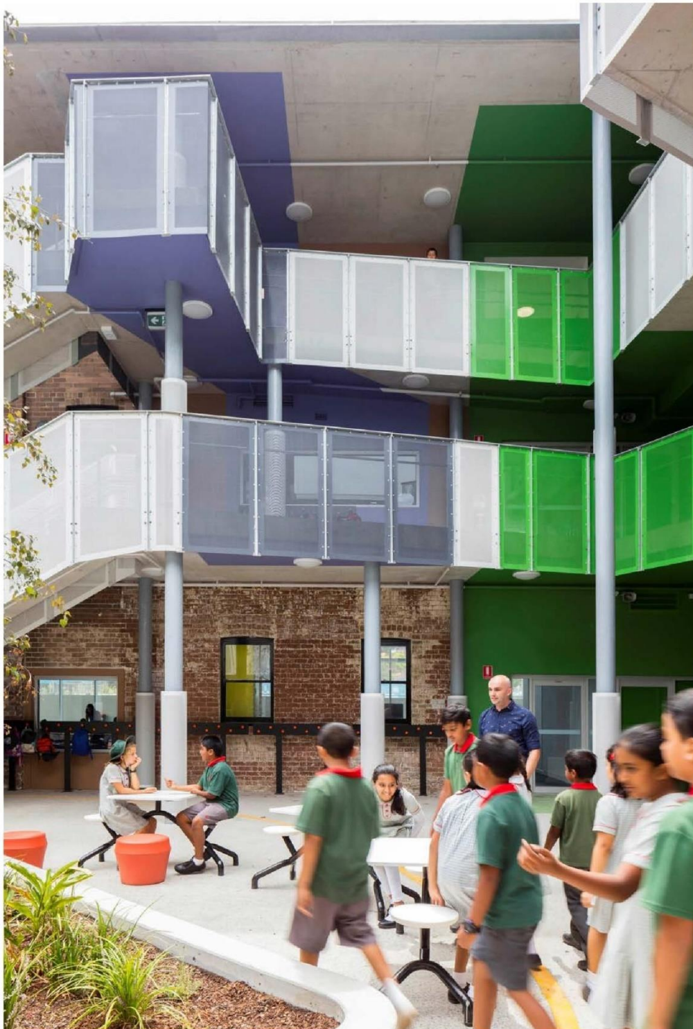
O'CONNELL STREET PUBLIC SCHOOL, PARRAMATTA Photo credit: School Infrastructure NSW
