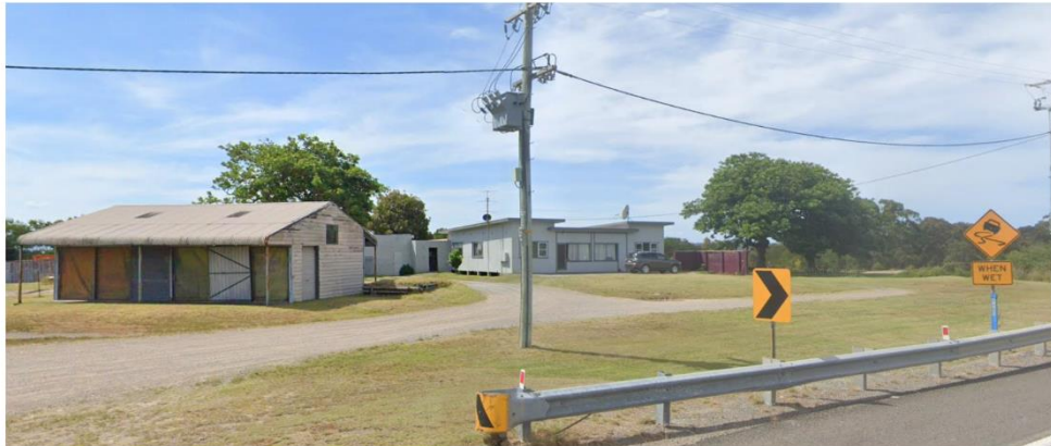
Figure 6: Buildings with separate entrance from Quarry, looking north east from Pacific Highway (Source: Google Streetview)
