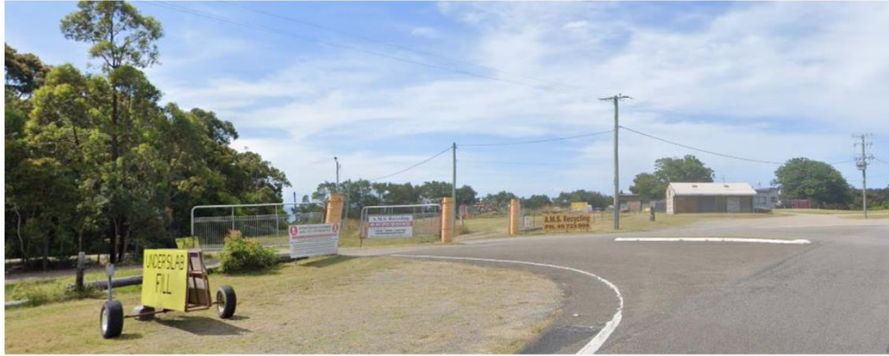
Figure 4: View of existing quarry entrance at the subject site, looking north east from Pacific Highway (Source: Google Streetview)
