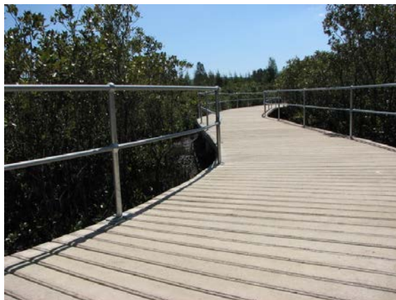
Photo 5: Example of an elevated pedestrian / cycleway
