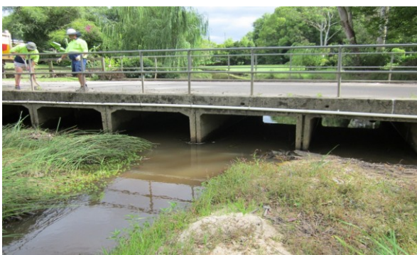
Photo 2: Debris under Tall Timbers estate access road
