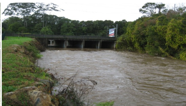
Photo 3: Flood downstream of Pacific Highway (2012)
