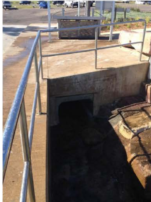
Figure 10: Western stormwater culvert entering Terrigal Haven Beach from carpark and Terrigal Haven streets near the dog off-leash park.
