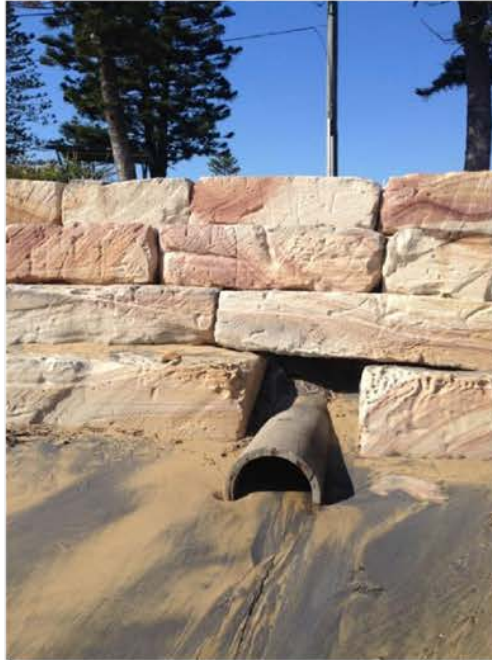
Figure 8: Central stormwater drain entering Terrigal Haven Beach from carparks, streets, oval and beach shower.
