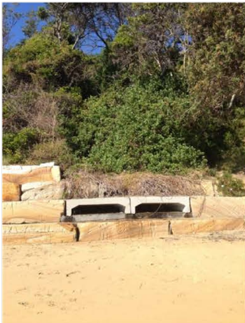
Figure 9: Eastern stormwater culverts entering Terrigal Haven Beach from Scenic highway and residential areas.
