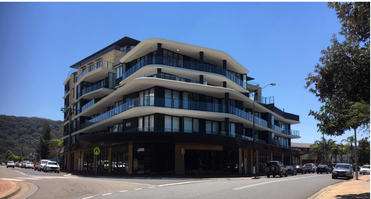
Figure 7 – Photograph mixed use development across the road from Mantra – 49 The Esplanade CDA (November 2019)
