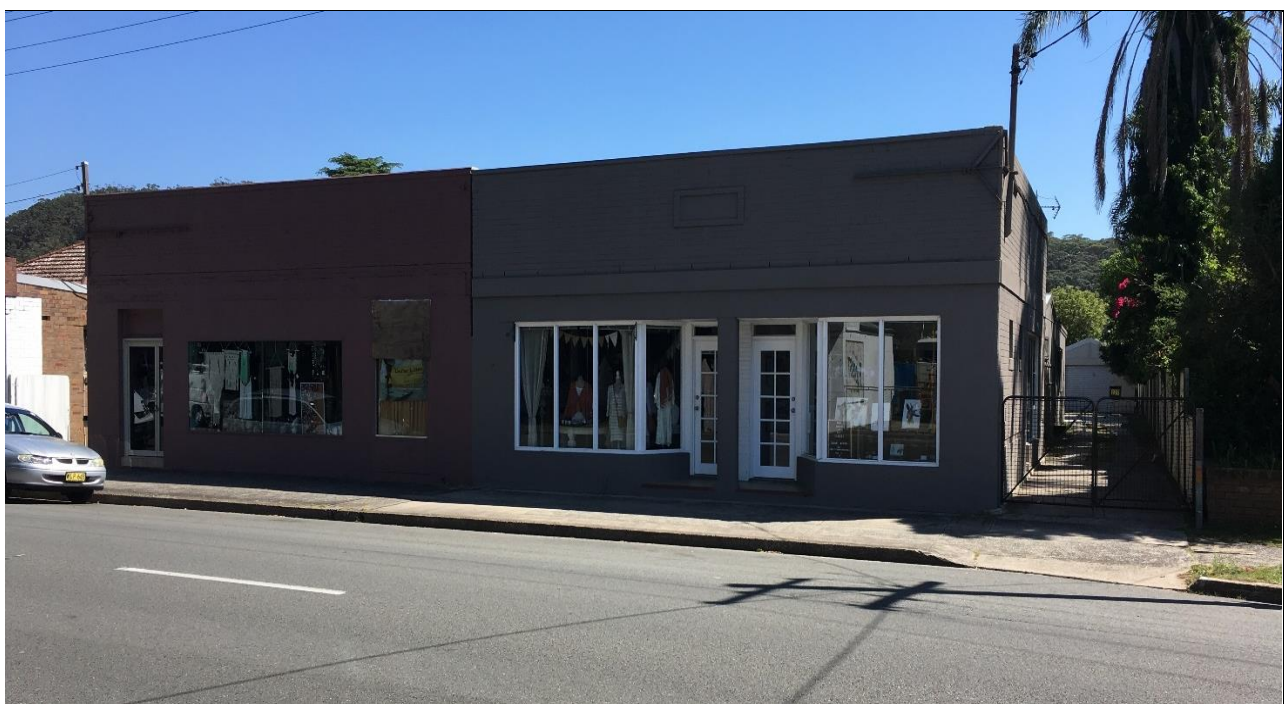
Figure 5 – Photograph of the site from the street
