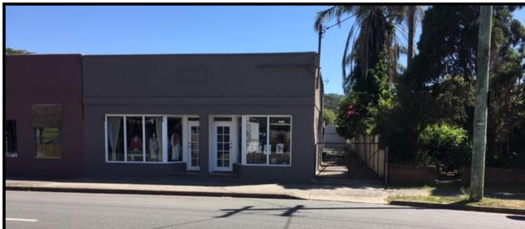
Figure 17. The zone interface at the eastern end of the R1 strip – No.227 Ocean View Rd. CDA Nov 2019
