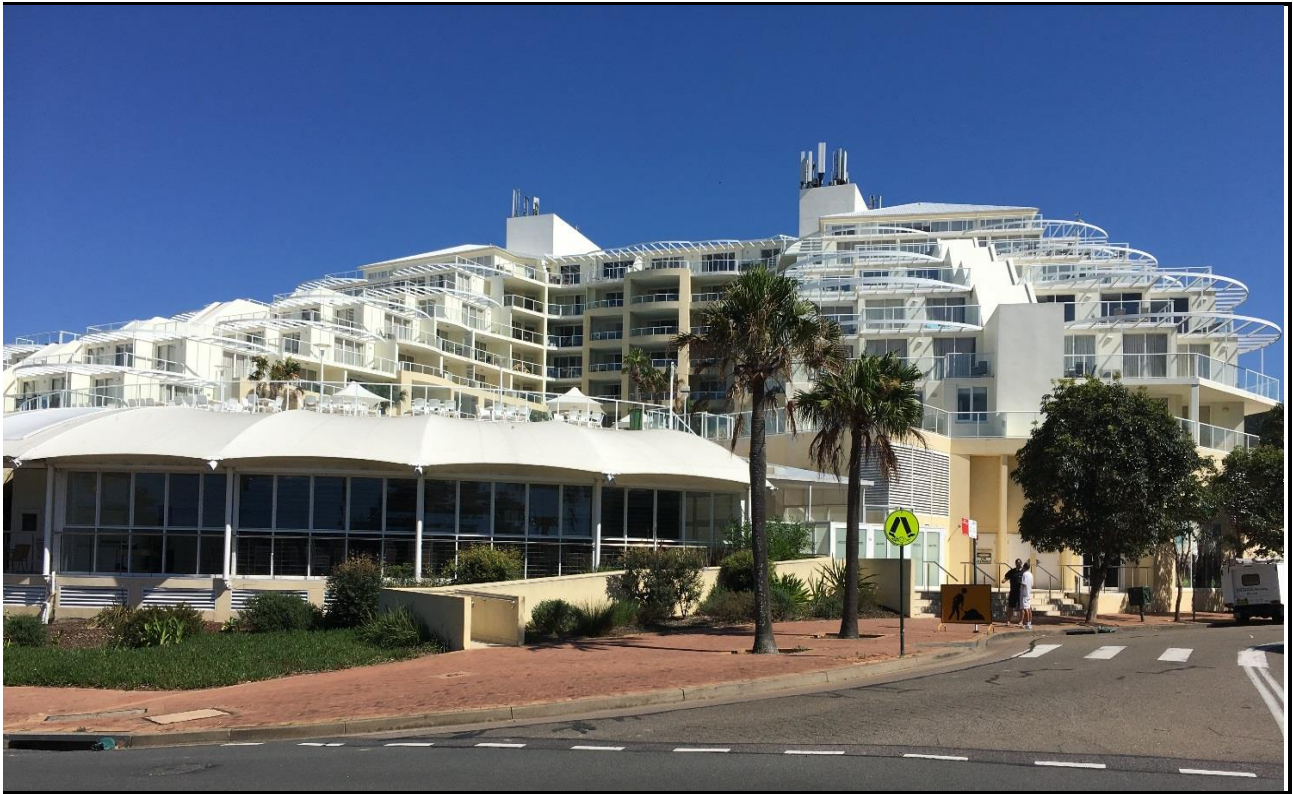
Figure 8 – Photograph of the Mantra apartments – located nearby
