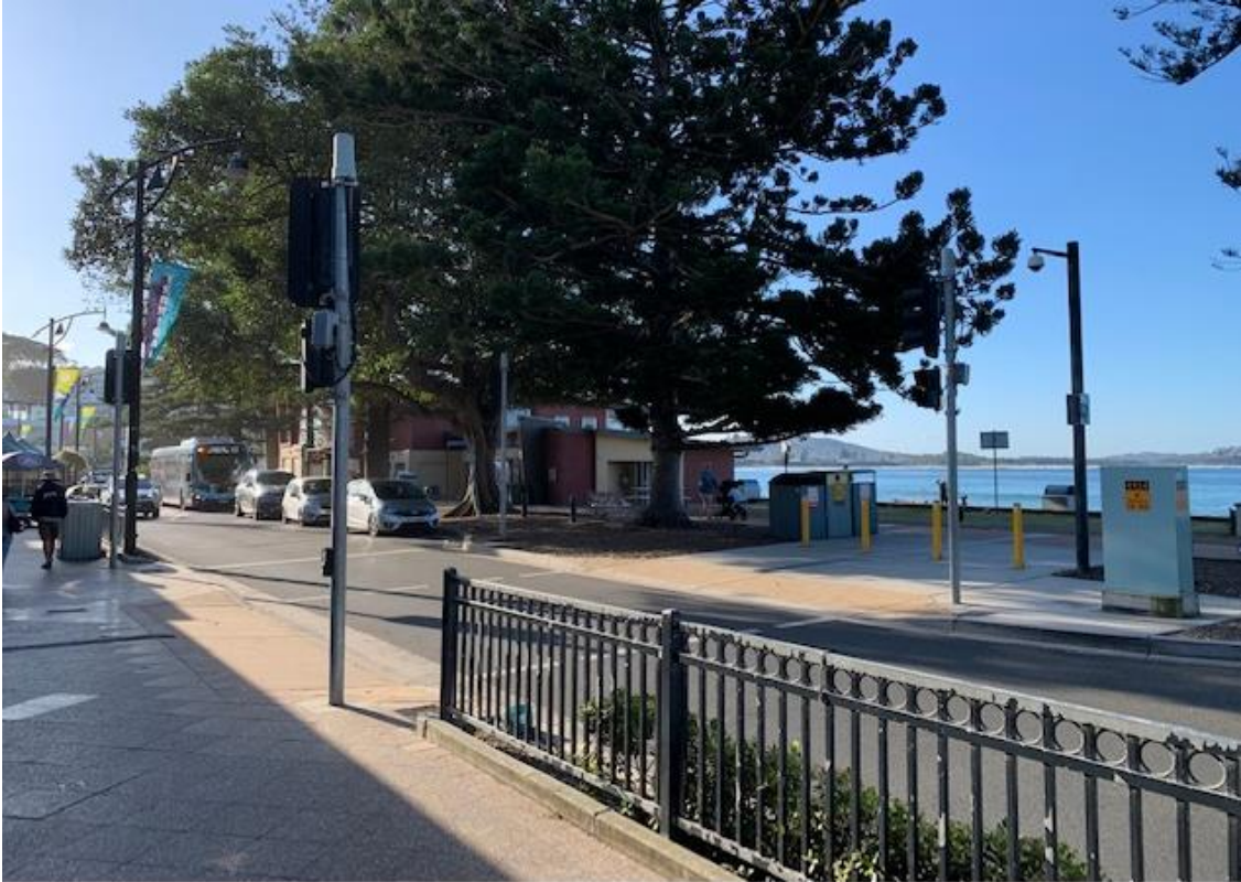
Photograph 1 - View of existing southern end of club from opposite side of Terrigal Esplanade
