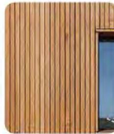
7 Proposed timber battens cladding to front face of wall
