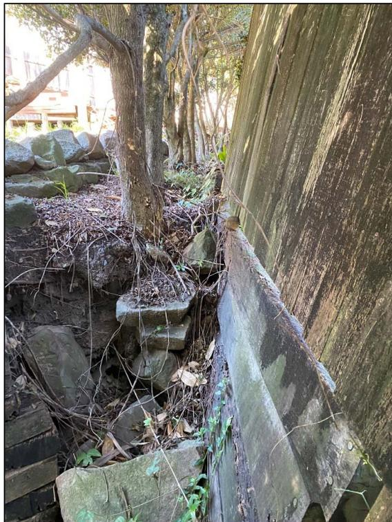
Photograph P3 – View of failed timber retaining wall along western boundary
