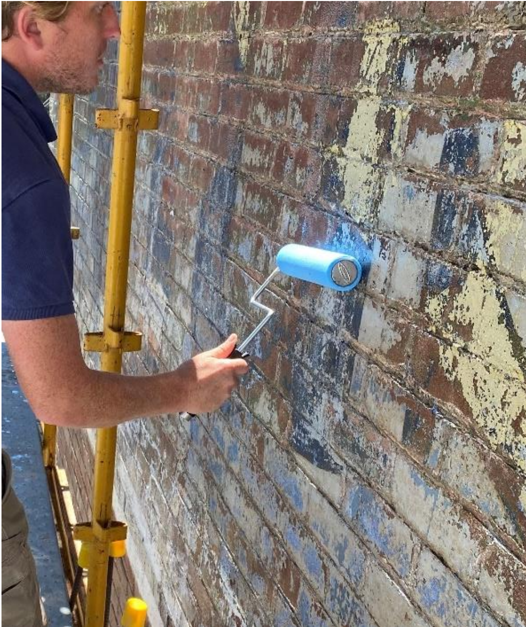
Image 11: During Treatment, surface coating, 13 th October 2020
