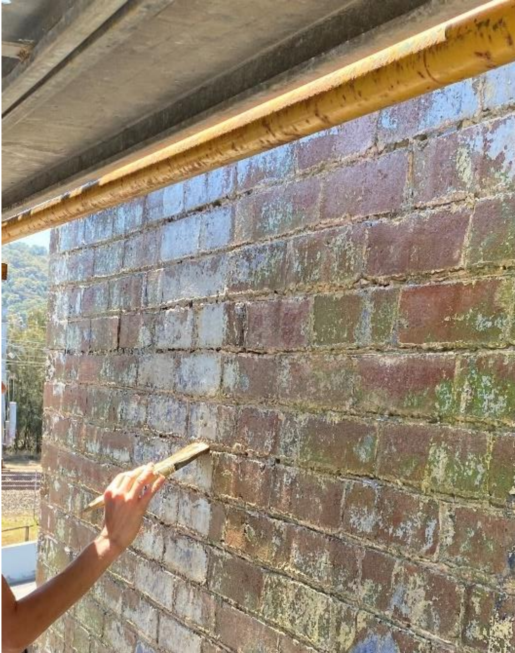
Image 10: During Treatment, consolidation, 12 th October 2020
