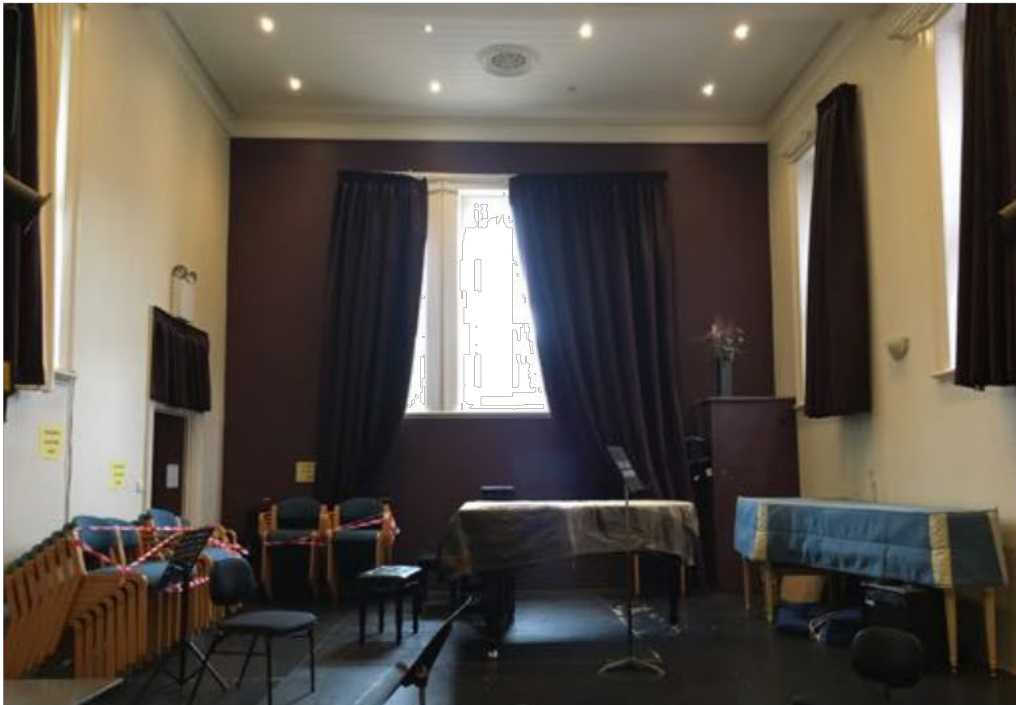
Figure 12: Subject Site: Existing Robert Knox Hall, Western facade.
