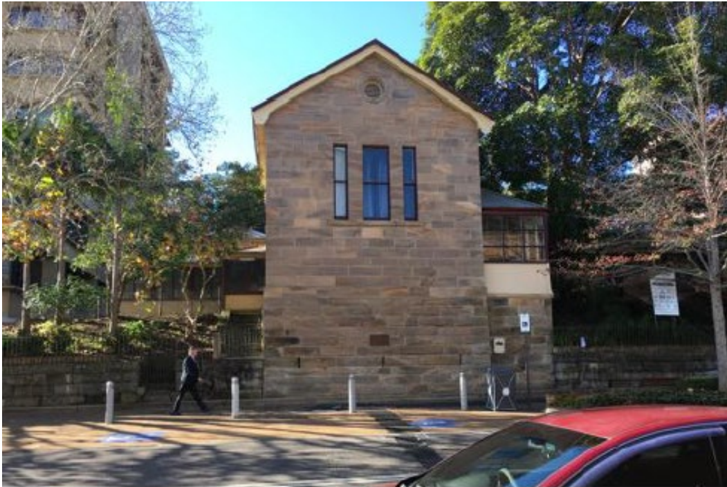
Figure 2- Existing Building viewed from Mann Street.
