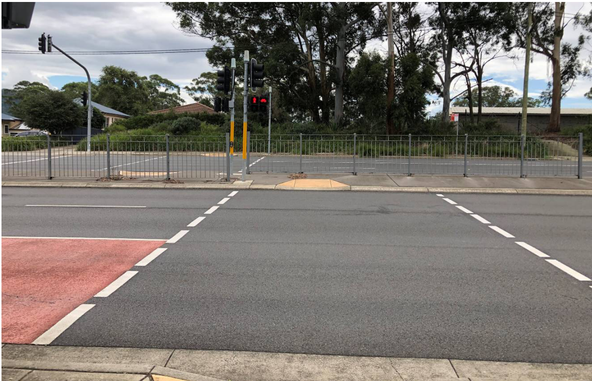
Photograph 5 – Split signalised pedestrian / bicycle crossing / refuge fronting the site.
